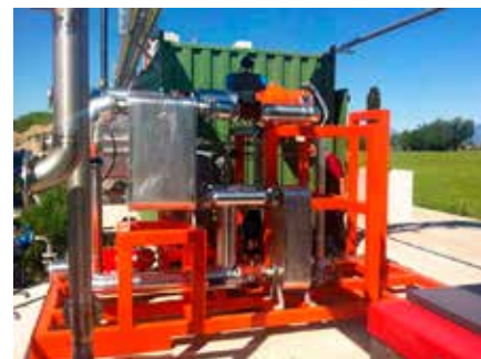
S. Pietro in Gu (Padua) - Heat recovery from cooling jackets and exhausts of biogas-fueled engines
