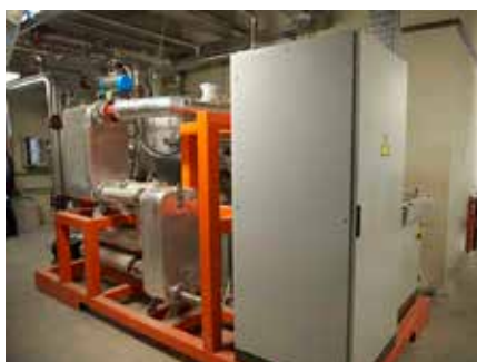
Meran (Bozen) - Heat recovery from cooling jackets and exhausts of gasifiers and syngas-fueled engines
