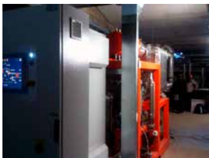
Rome - Heat recovery from cooling jackets and exhausts of gasifiers and syngas-fueled engines
