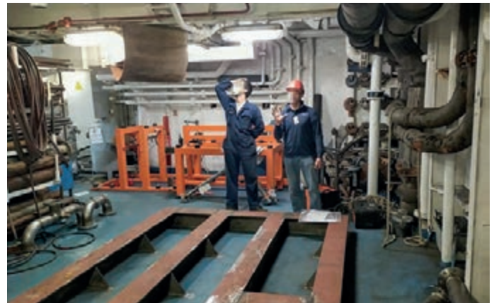
The narrow technical space where the skid is going to be hosted and its I-beam support frame, welded to the floor
