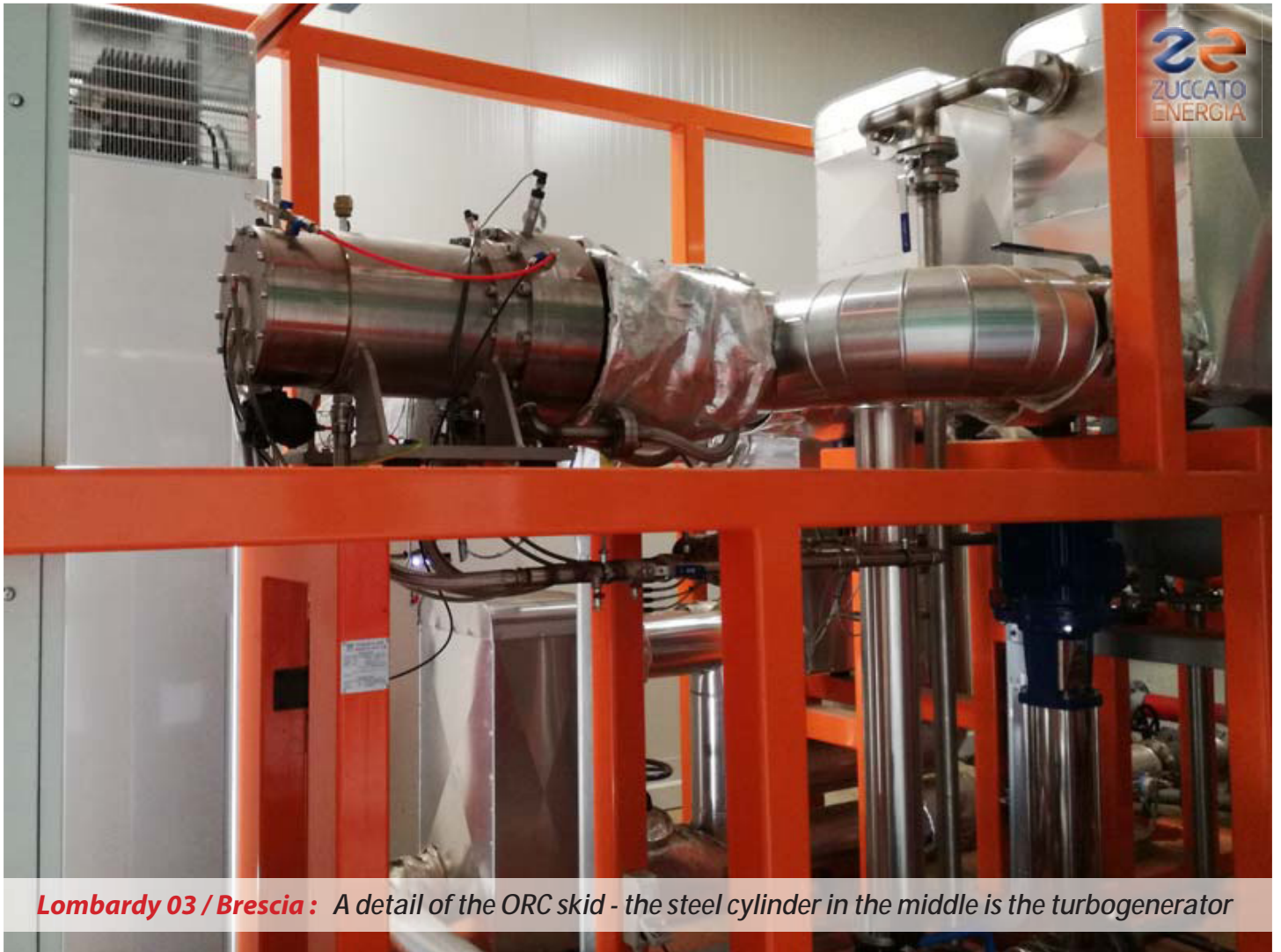
Lombardy 03 / Brescia: The ZE-150-LT ORC power generation module, seen from the control panel side
