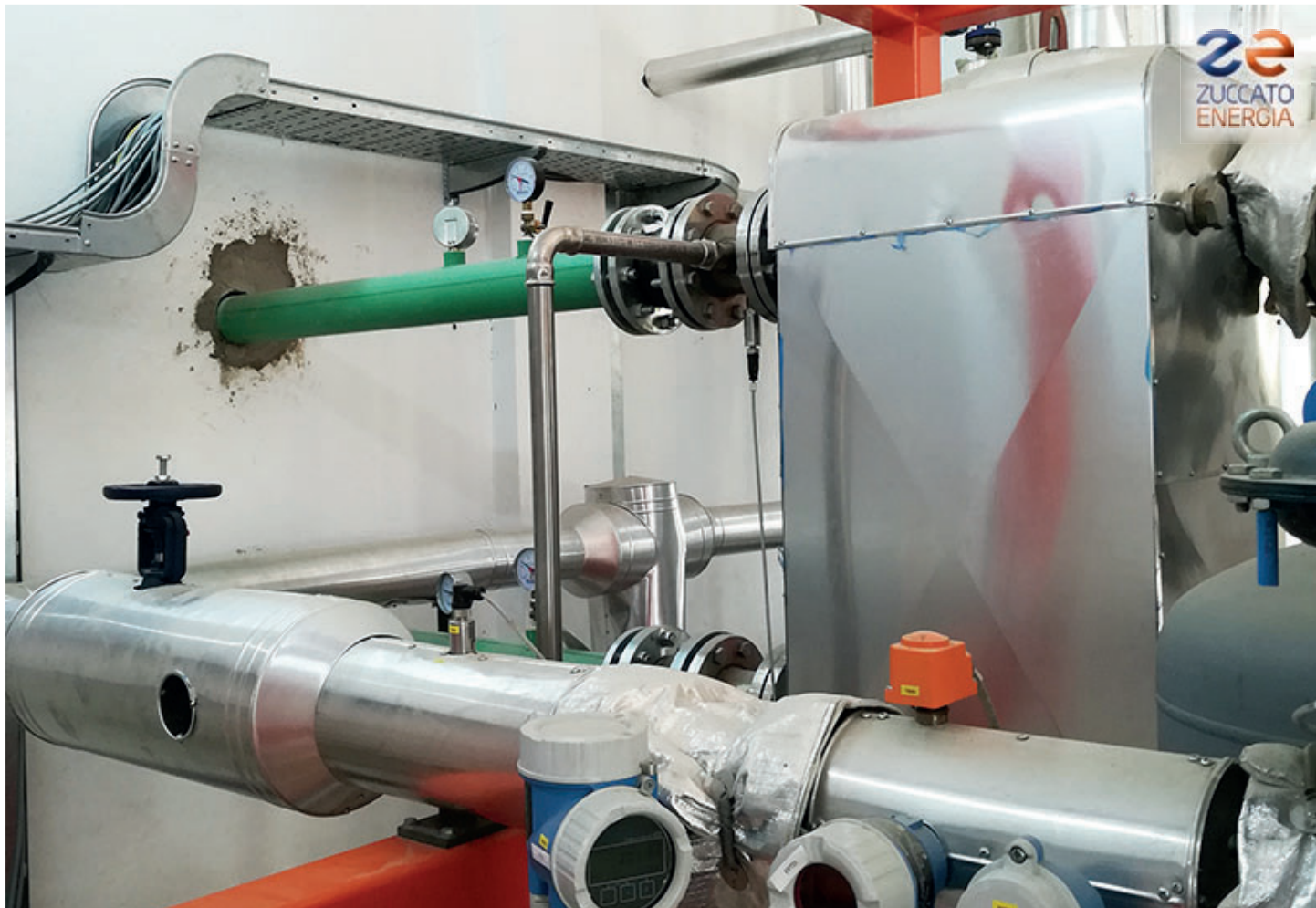
Tunisia 01: The heat exchangers. This was the first plant by ZE using live saturated steam as a vector fluid.
