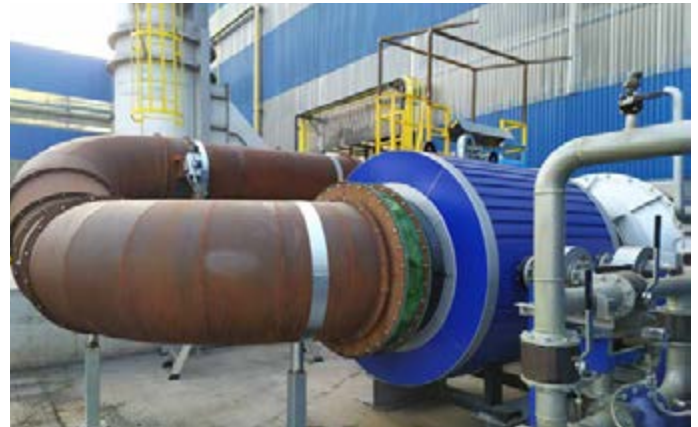
The heat exchanger (blue) installed on the fume gas line
