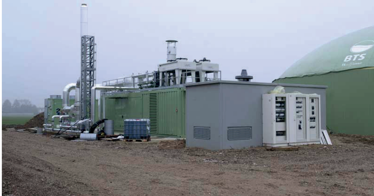
Lombardy 01 / Mantua: Overview of fermenters, motors and containerized ORC ZE-50-ULH module.
