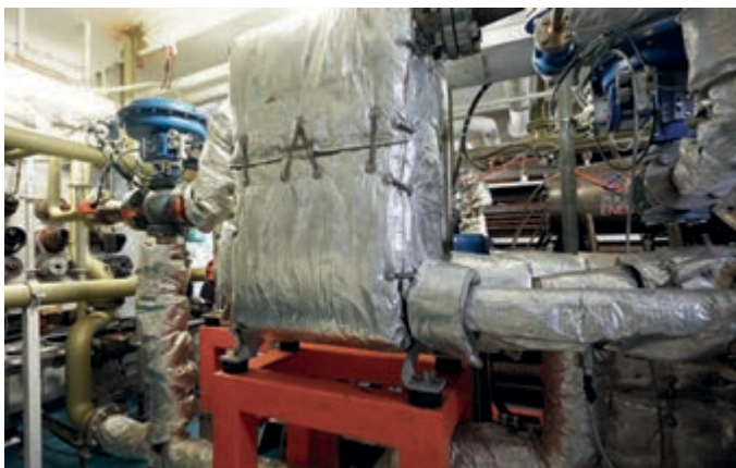
The ZE-100-LT skid in place. L to R: the blue 3-way valve, the main heat exchanger and the turbogenerator (far right)
