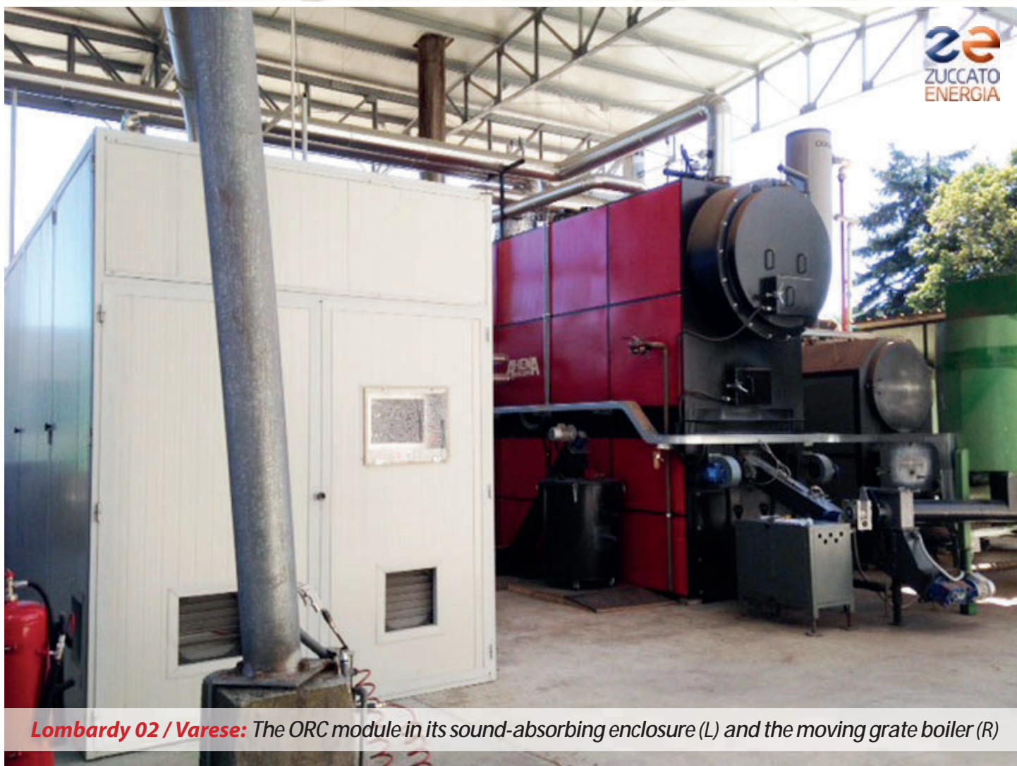
Lombardy 02 / Varese : Plant overview: ORC module (white), boiler (red) , wood chip storage and loading (green)
