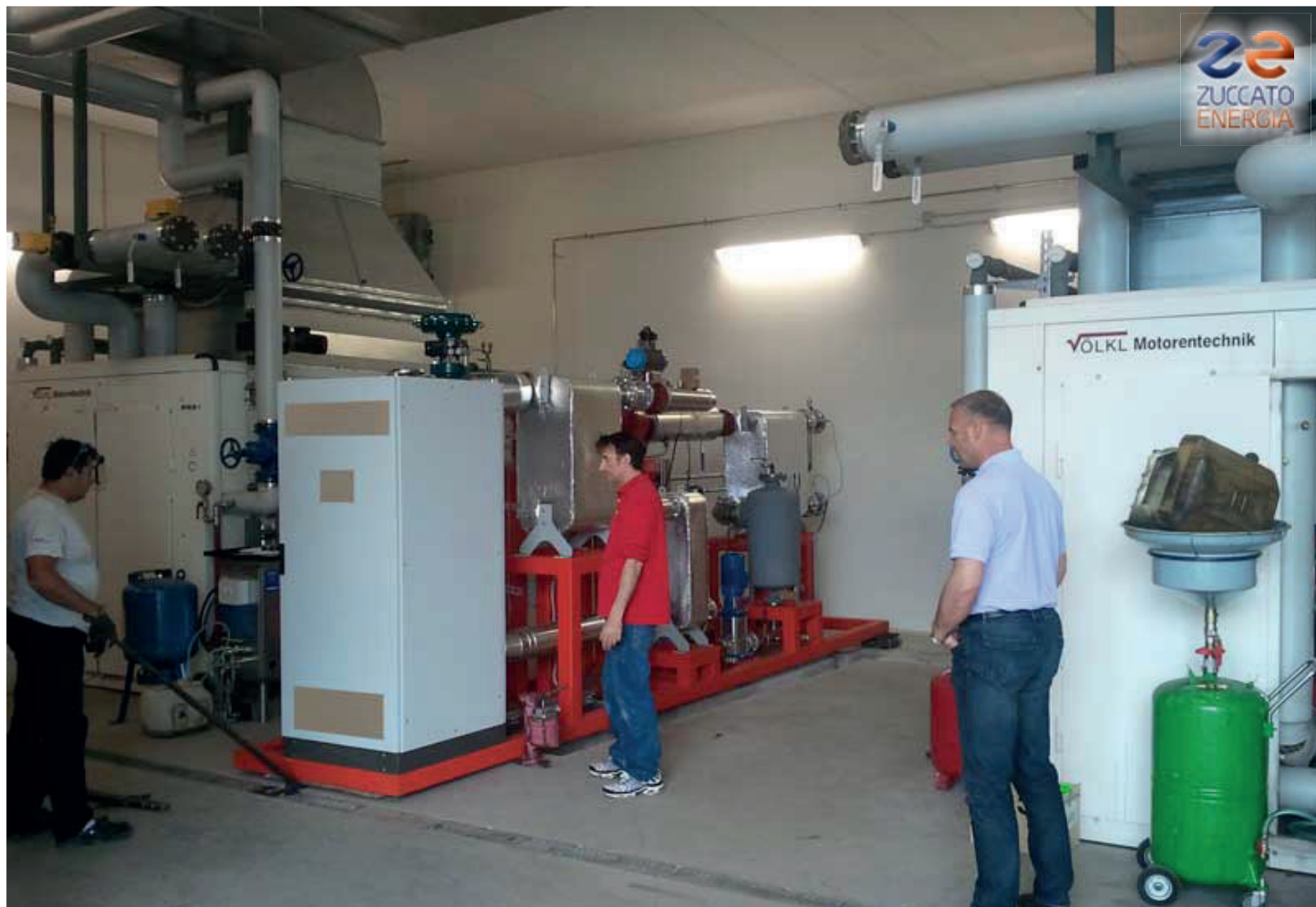
South Tyrol 04 / Bozen: The first of the two ZE-50-ULH ORC modules on its custom skid during installation.
