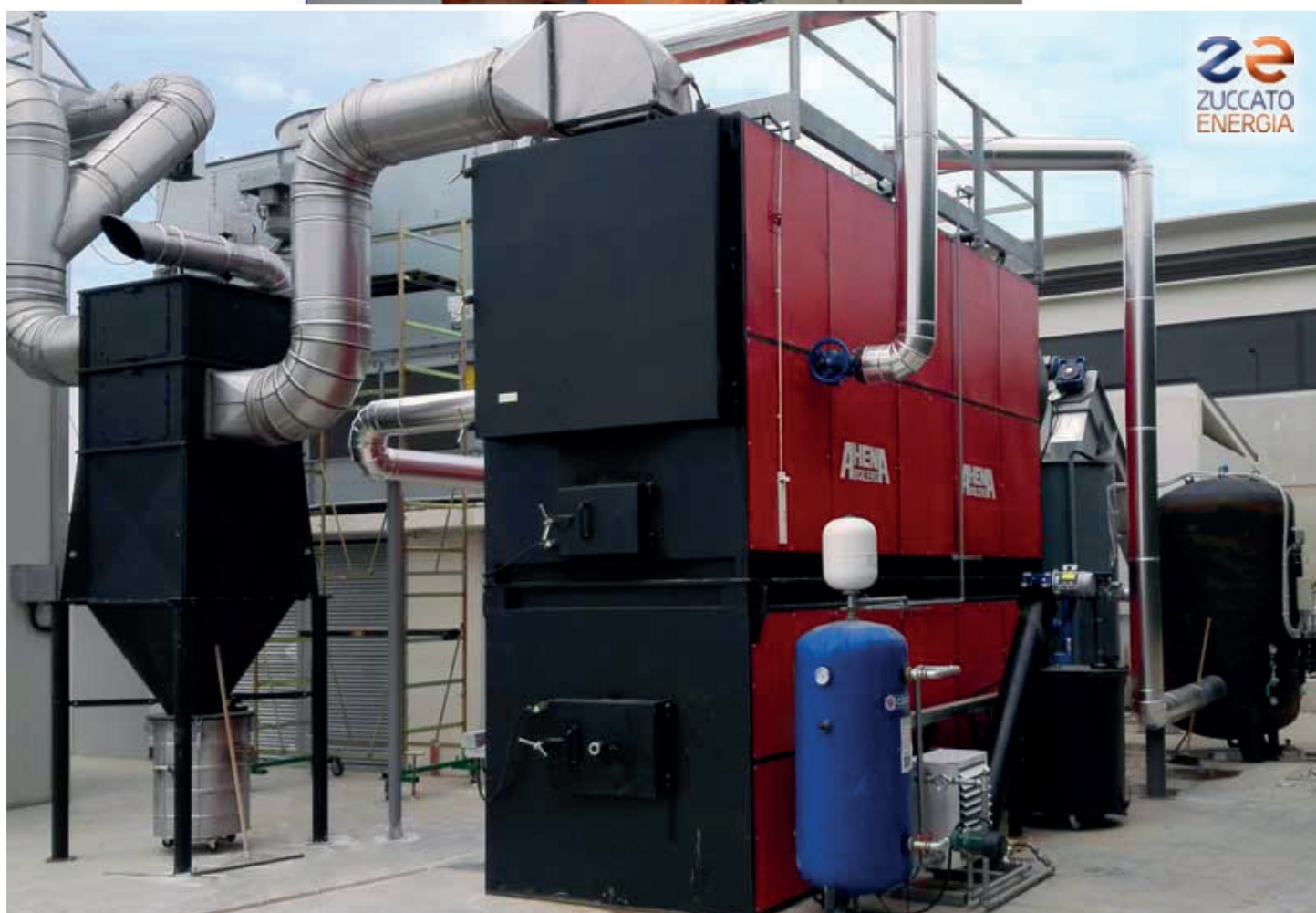
Sicilia 01 / Ragusa : The 1.3MWt moving grate boiler , fed with wood chips (fruit crate production waste)
