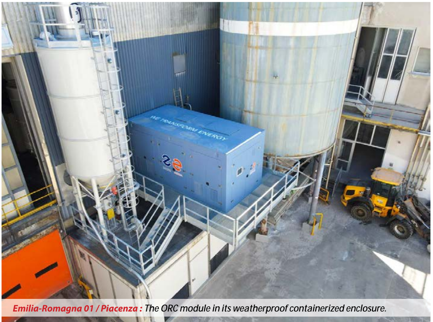
Emilia-Romagna 01 / Piacenza : The ZE-200-LT ORC module before installation
