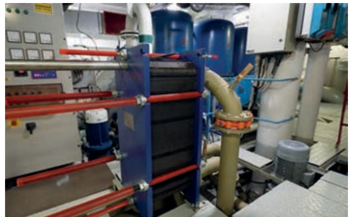
The inspectable heat exchanger used to exchange heat between the cold side condenser of the plant and the sea
