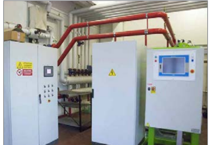
The plant control panels
