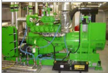
The vegetable oil engine in more detail
