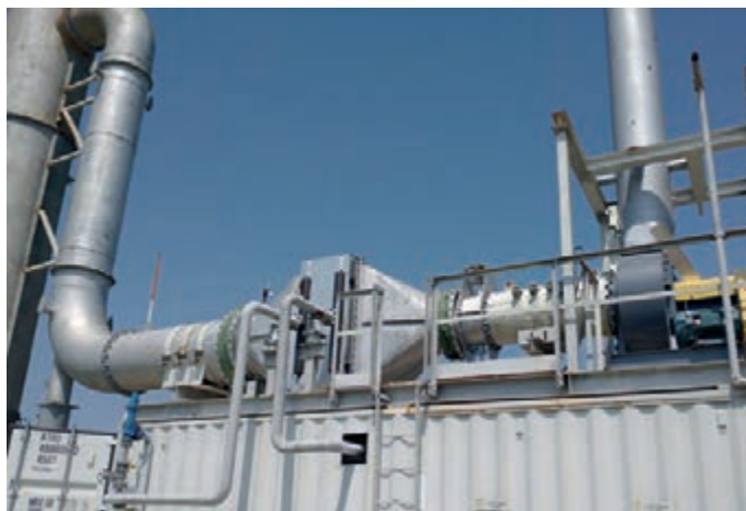
A detail of the primary heat exchanger. Hot gases are drawn from the combustor on the left and pass thru the exchanger
