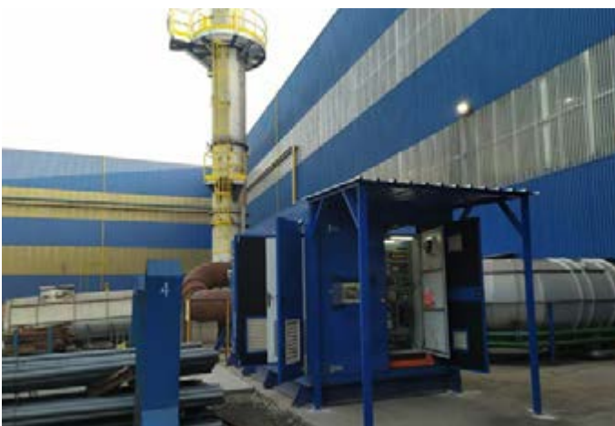
An overview of the ORC ZE-200-LT from the side
