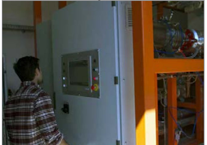
The ORC skid control panel
