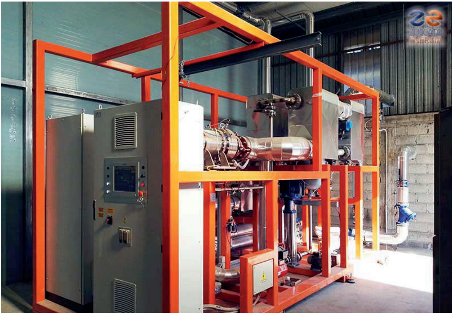
Calabria 01 / Cosenza : The ZE-175-LT ORC module in its place, seen from the control panel side
