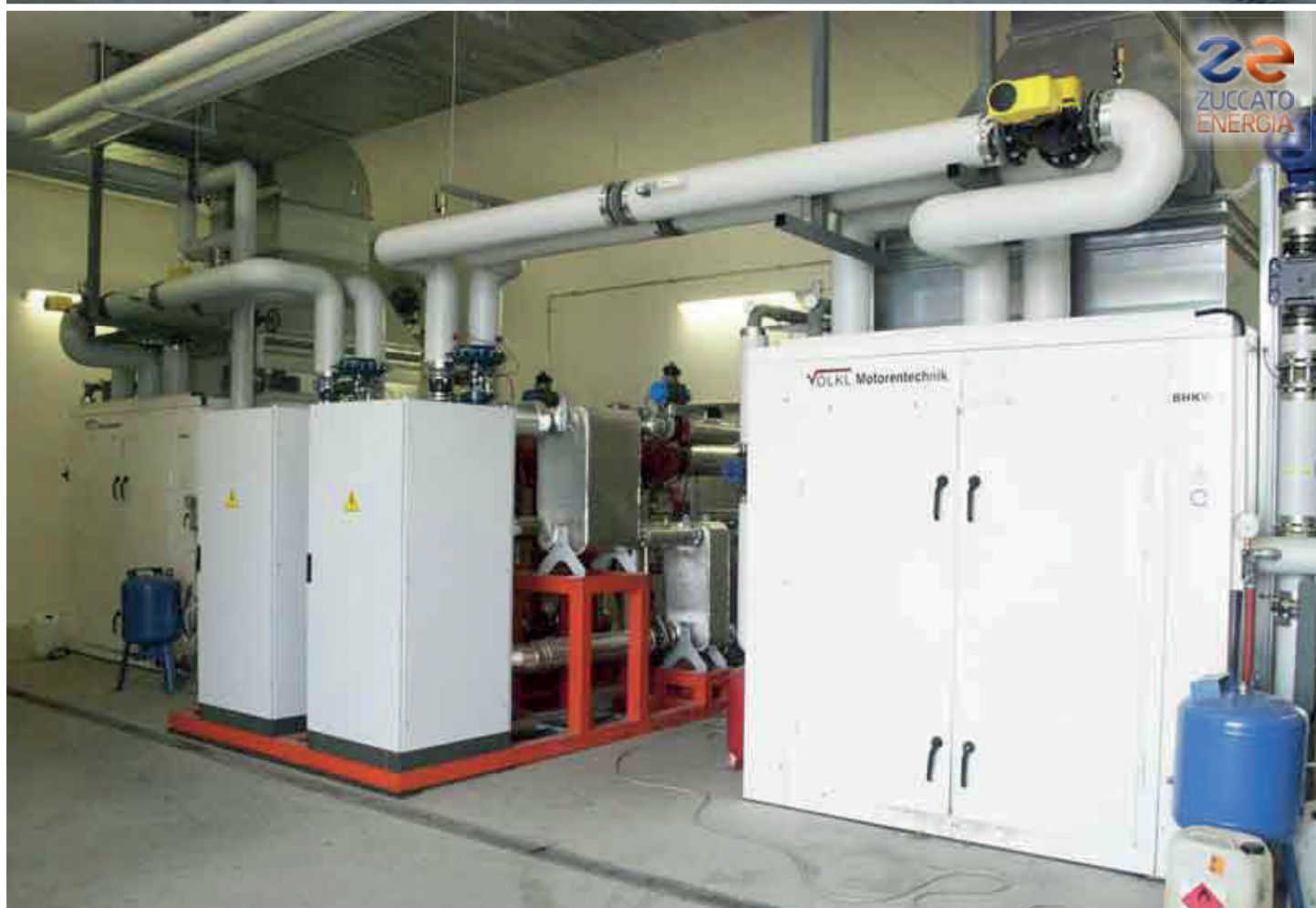
South Tyrol 04 / Bozen: The complete ORC installation modules linked by the motors it recovers heat from.
