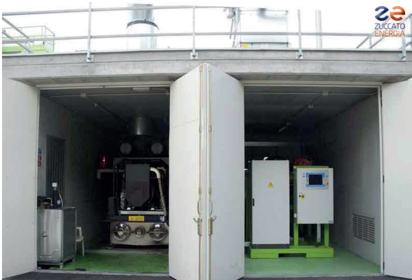
South Tyrol 01 / Bozen: The vegetable oil engine (L) and the ZE-50-ULH module (R) in their concrete shelter.
