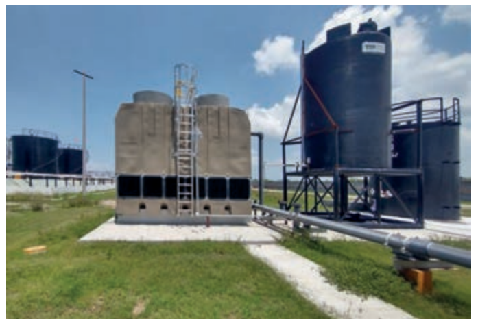
The evaporative cooling tower of plant B. The black vertical tanks on the right contain the cooling water supply.
