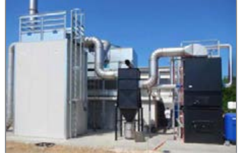
R to L: boiler, dust trap and and ue gas treatment system
