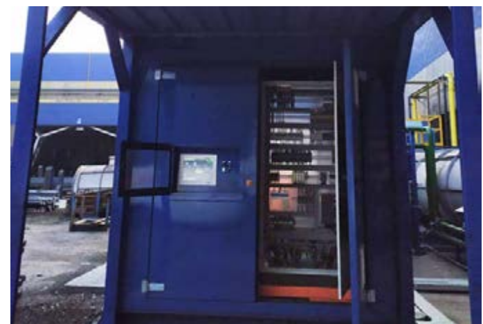
Access area to the ORC control panel and electronics
