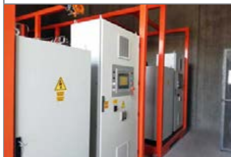
The control panels for the ORCs
