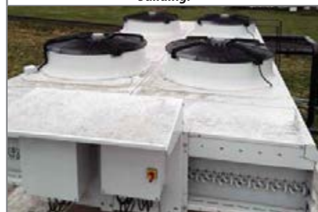
A detail of the dry cooler placed on the roof
