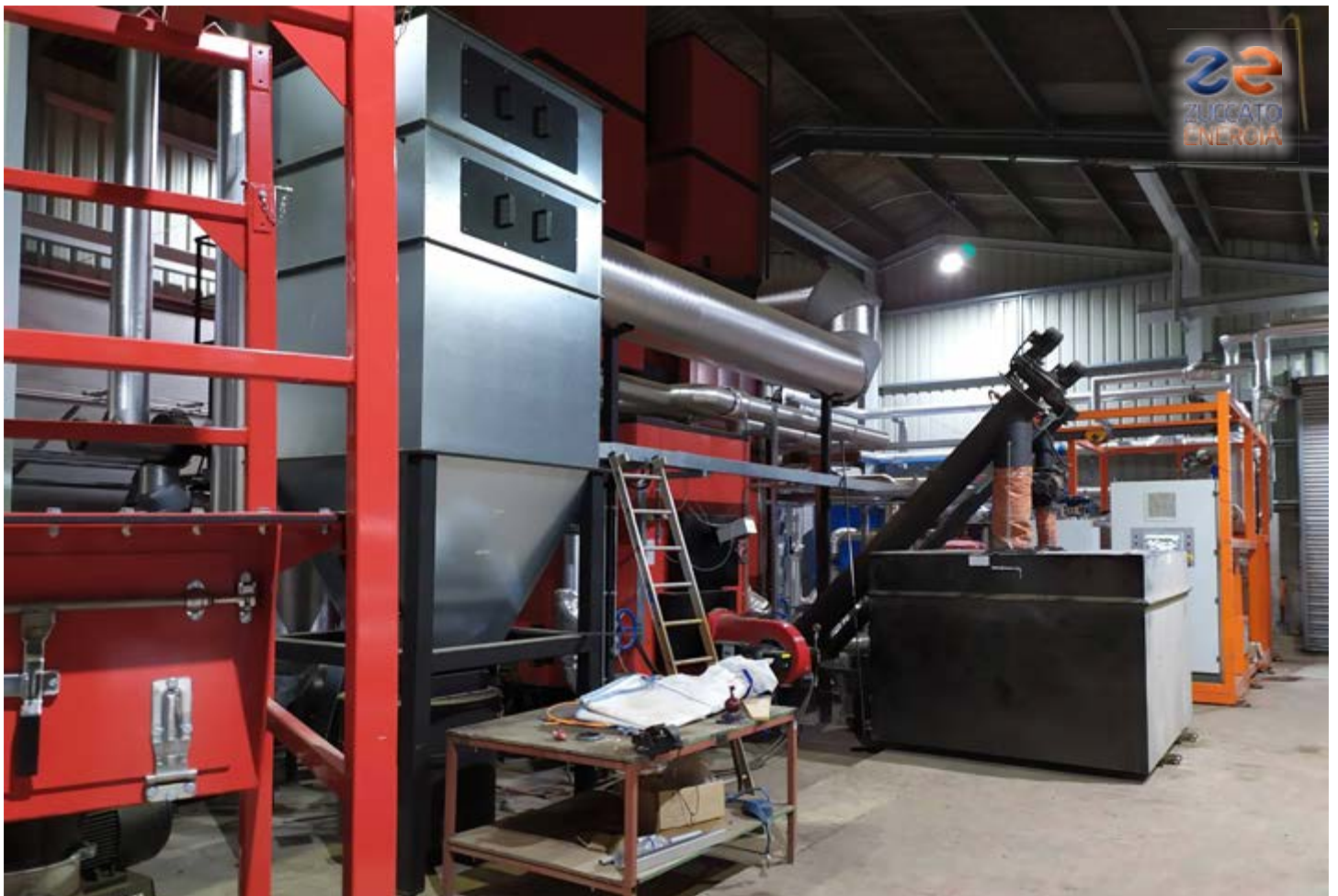
United Kingdom 01 : The Entire plant - chipper, loading hopper, boiler and ORC module
