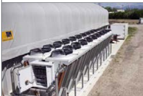
General view of the dry cooler
