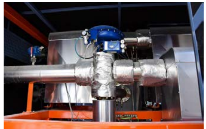
Three-way Diverter Valve
