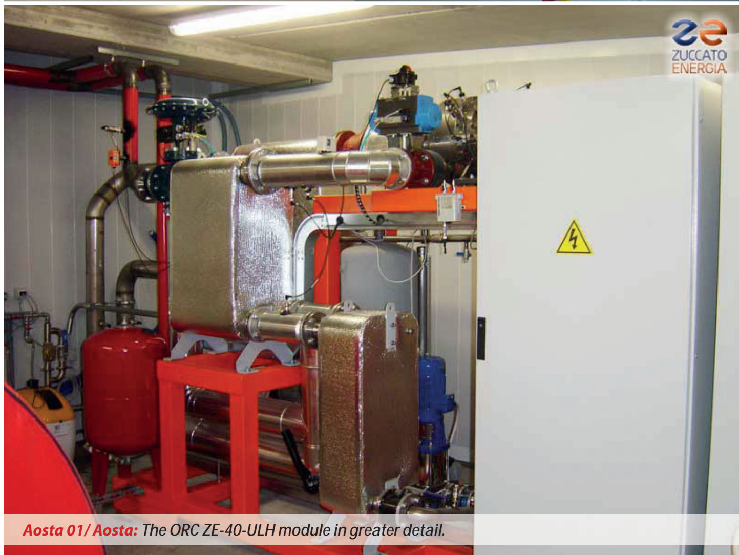
Aosta 01 / Aosta: General view of the boiler room - motor (green), thermal buffer (red) and ORC module (white)
