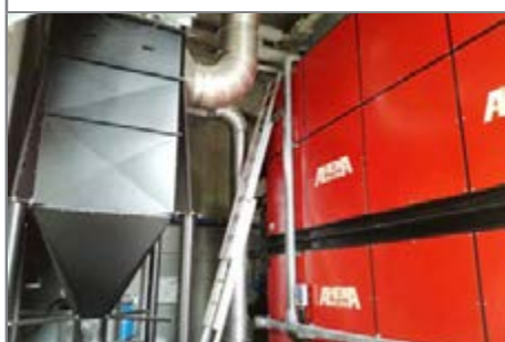
A detail of the boiler and its ash filter.
