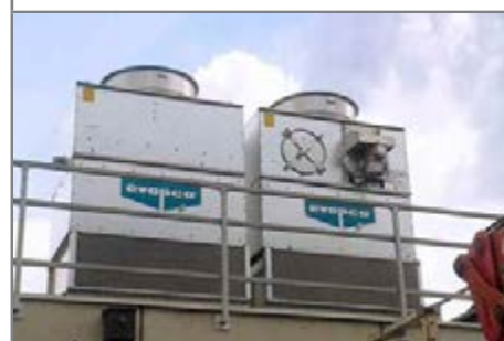
The cooling towers for the condensing stage.
