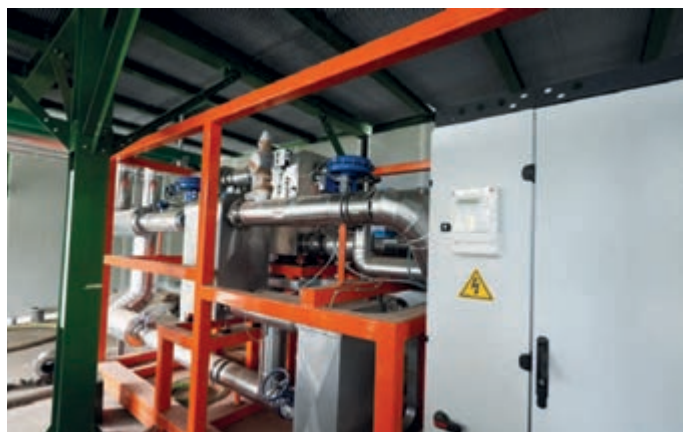
The ZE-200-LT skid in its place below the cooling system. The cabinets hosts electronics and local control panel
