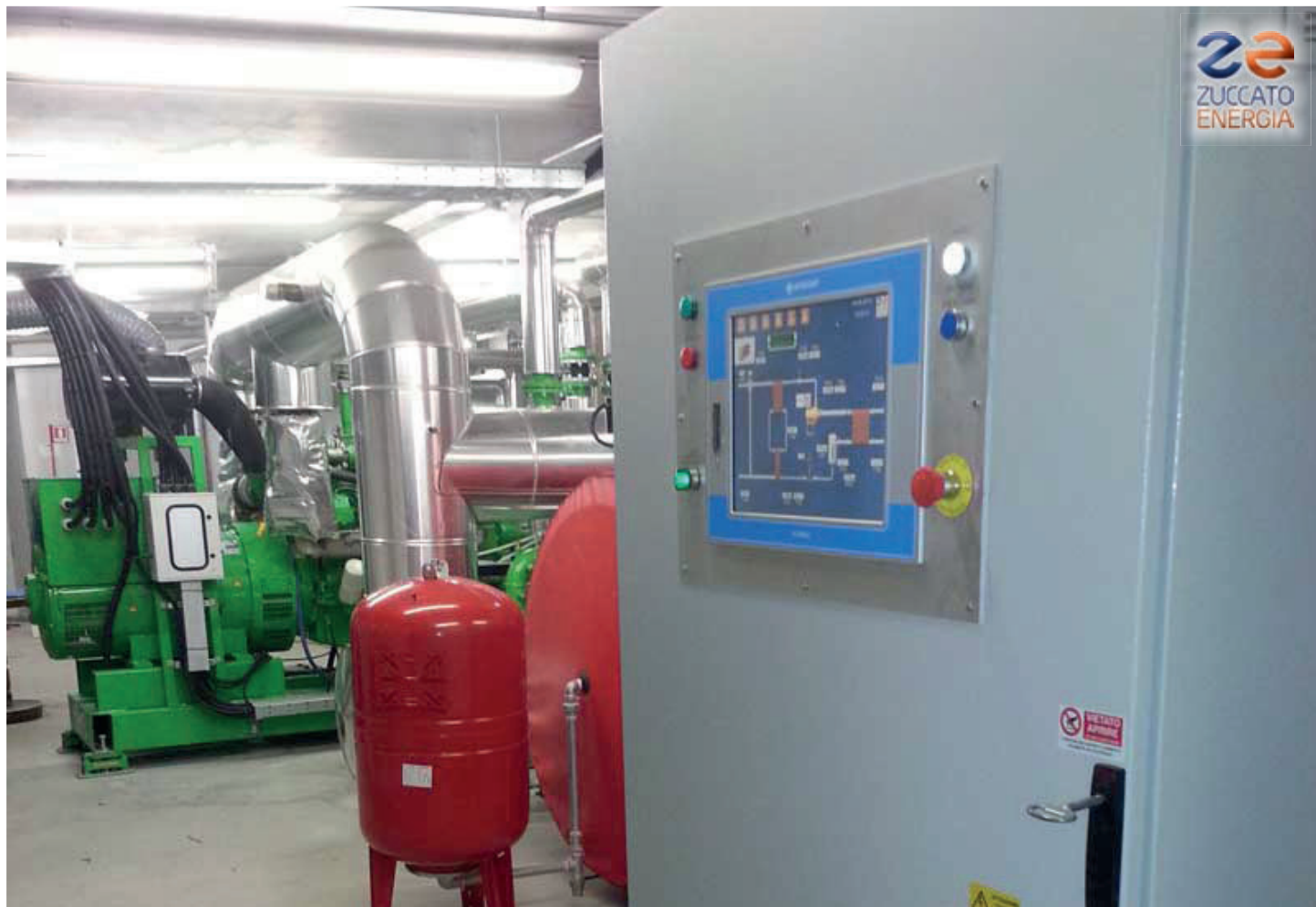
Aosta 01 / Aosta: General view of the boiler room - motor (green), thermal buffer (red) and ORC module (white)
