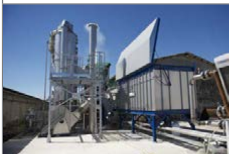
Fuel loading hopper and chimney
