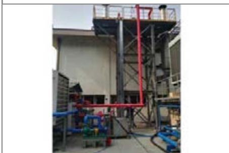
The hot-side piping conveying heat to the ORC. The heat exchanger is on the platform at the top
