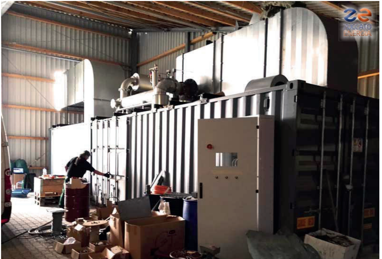
Germania 02 / Lower Saxony: The container hosting the biogas-fueled MAN genset
