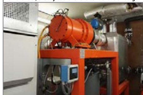
The ORC ZE-50-ULH skid in place inside the building.
