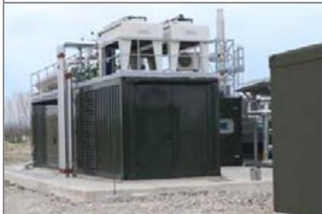
The container housing the biogas engine
