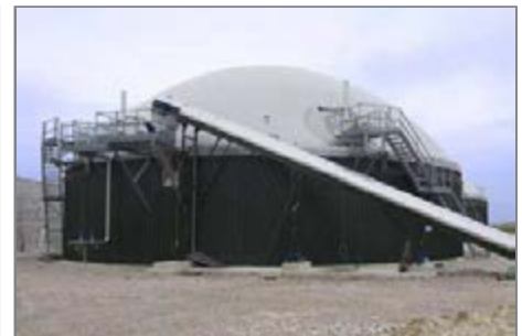
One of the fermenters with its loading auger
