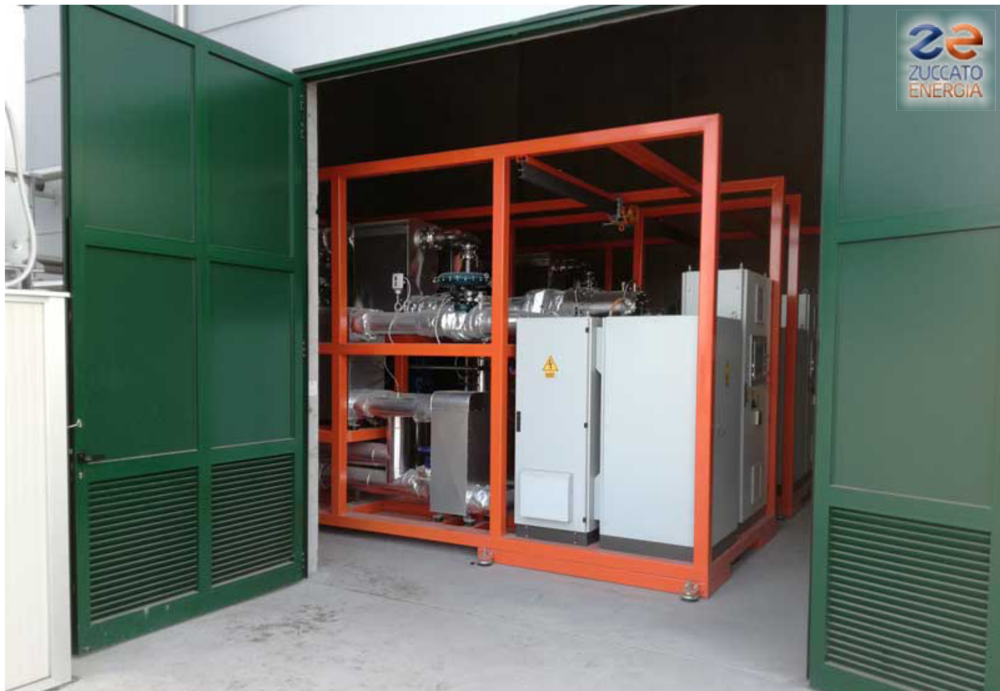
Veneto 04 / Padua: The two skid-mounted ZE-100-LT Organic Rankine Cycle modules in their room
