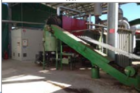
Detail of the wood chip conveyor to the boiler. On the bottom the skid.
