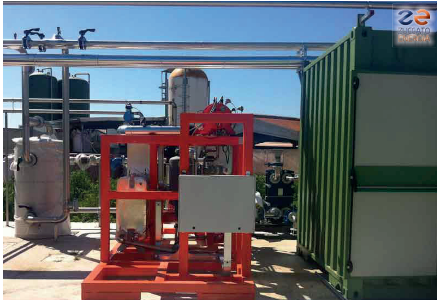
Veneto 02 / Padua: The ZE-50-ULH Organic Rankine Cycle module seen from the front.
