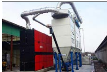
The boiler (left) and the fuel gas treatment plant
