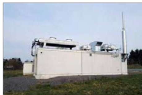
The east side of the prefab. On the roof, the dry cooler of the condensation stage.
