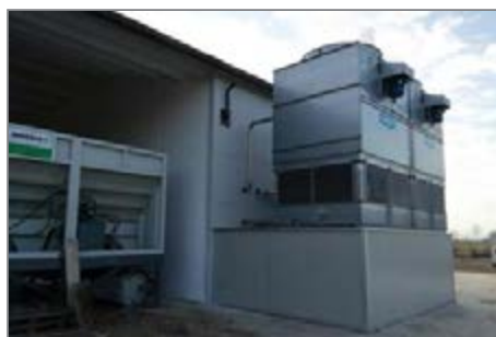
The evaporative cooling tower.
