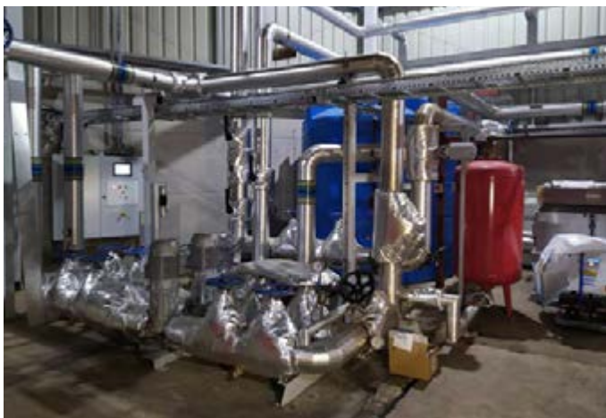
The boiler preheating system and part of the water loop.
