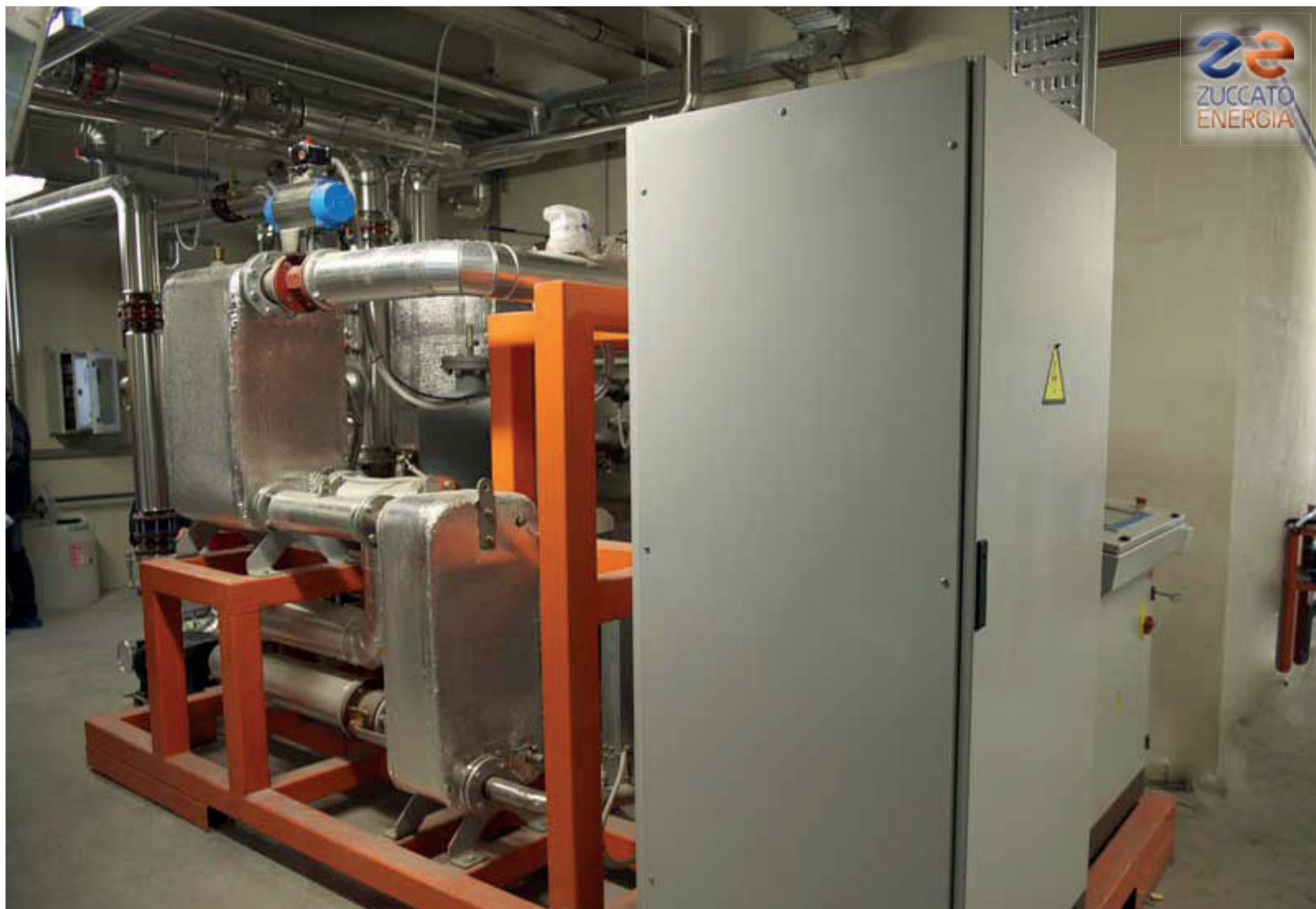
South Tyrol 03 / Meran: The ZE-50-ULH ORC module at the customer's site, viewed from the side.
