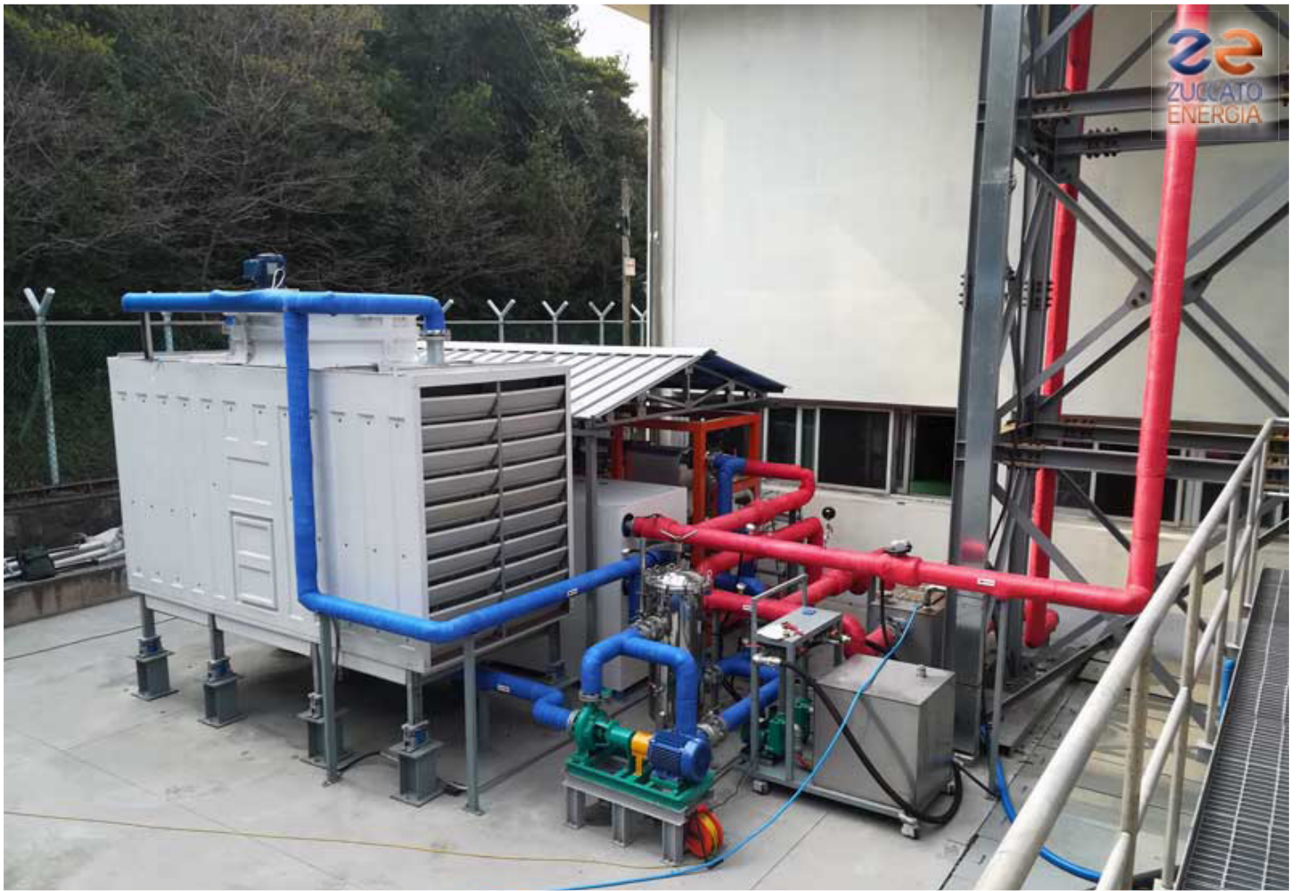
Korea 01 : The cooling tower and the awning hosting the ZE-40-ULH ORC power generation module
