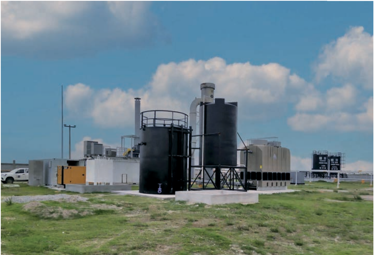
Mexico 01c / Veracruz : Plant C, seen from the rear . The yellow cabinet hosts the start-up generator.
