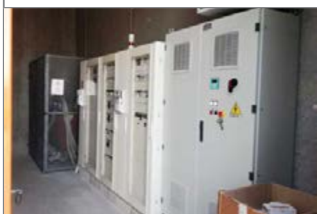
The mains grid interface panels.
