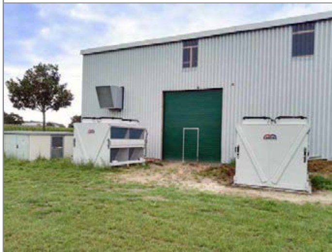
The entrance door to the shed and the dry coolers serving the condensation stage
