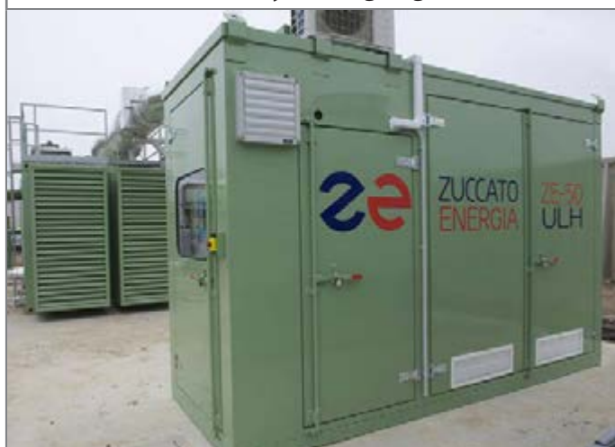
The right side of the containerized ORC module.
