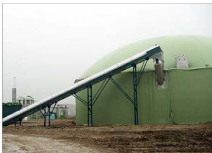
The slurry loading auger
