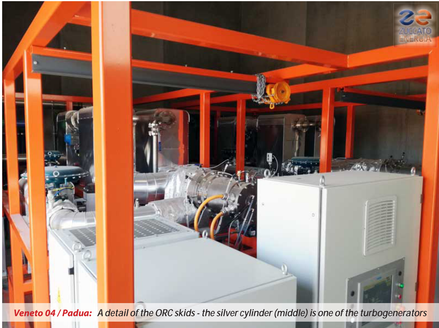
Veneto 04 / Padua: The two skid-mounted ZE-100-LT Organic Rankine Cycle modules in their room
