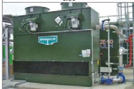
The cooling tower of the condensing stage
