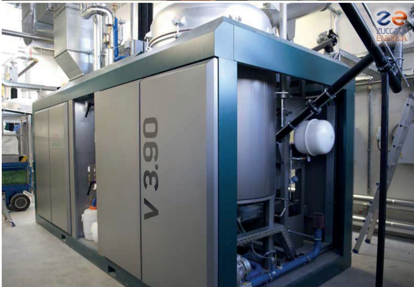
South Tyrol 03 / Meran: One of the gas inlets from which the ORC module recovers thermal waste.
