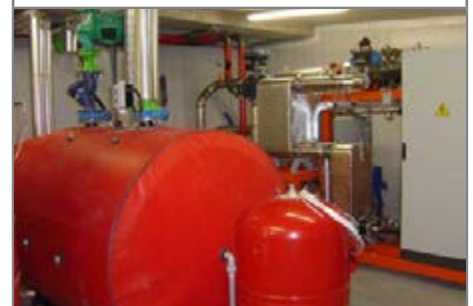
The thermal storage tank and the ORC module
