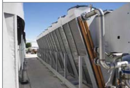
A detail of the dry cooler
