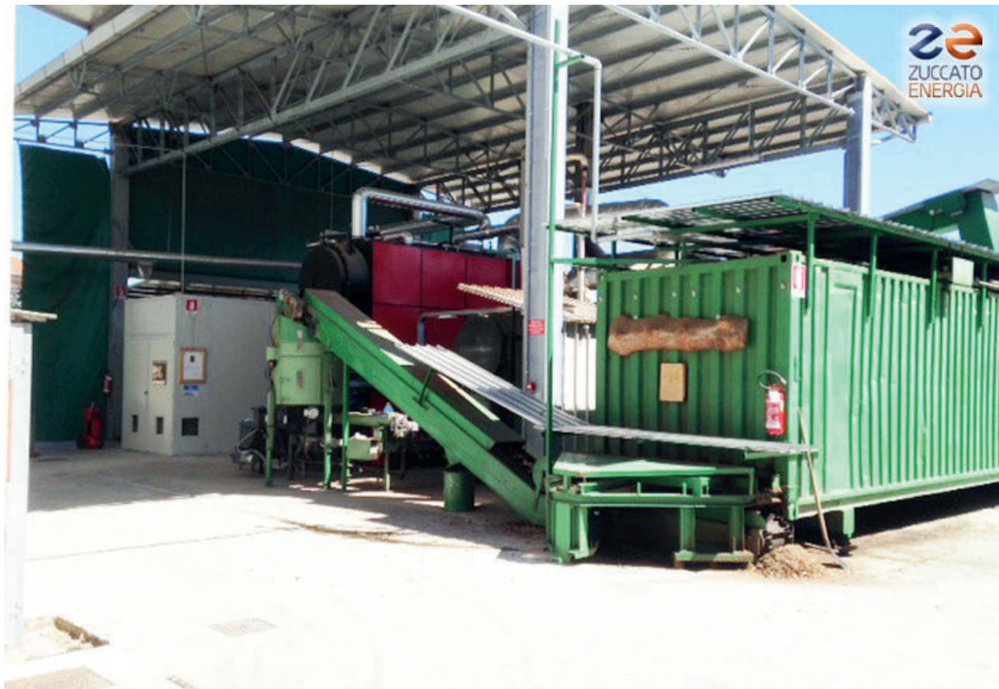
Lombardy 02 / Varese : Plant overview: ORC module (white), boiler (red) , wood chip storage and loading (green)
