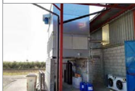
The tower base hosts the cooling water treatment system
