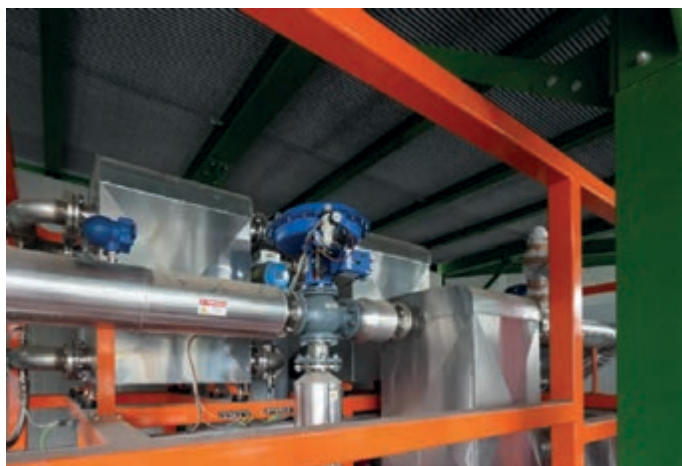
A detail of the heat exchangers aboard the skid and the blue 3-way valve that regulates the incoming heat flow
