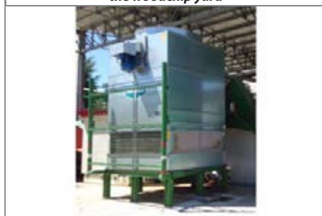
The cooling tower: some of the waste heat is used to dry the wood chips.
