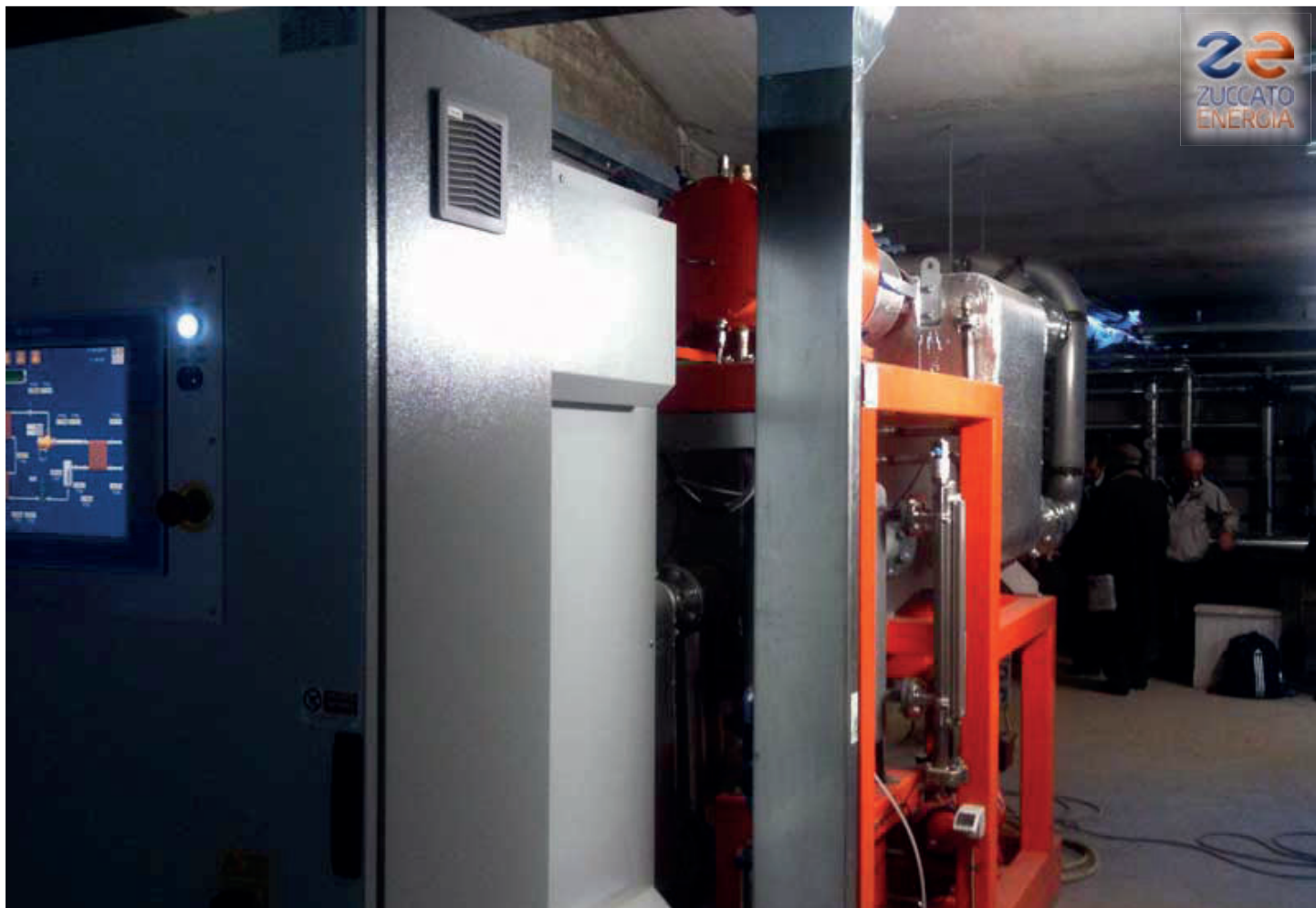
Lazio 01 / Roma: The ORC module in its underground room located under one of the movie theaters.
