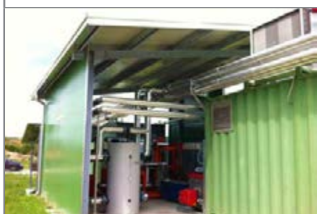
The ORC system under its awning
