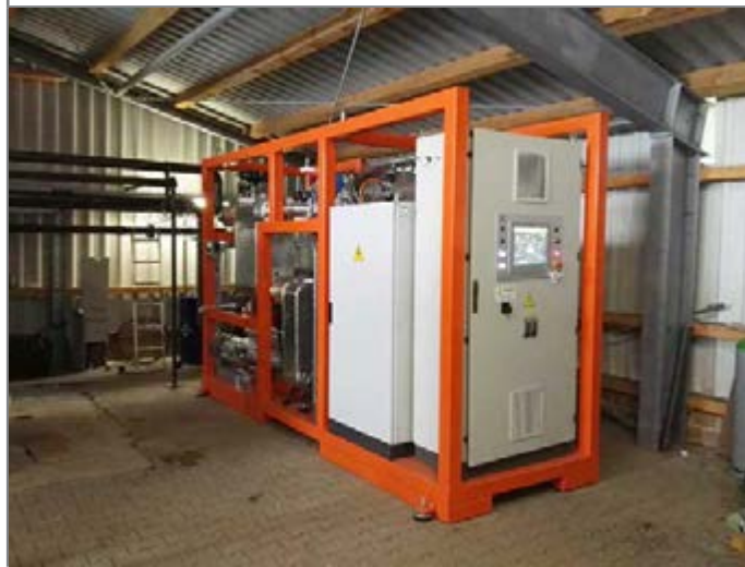
The ZE-40-ULH ORC module in place, seen from the control panel side
