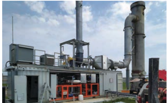
The ZE-200-LT ORC module inside its enclosure during installation. On the right, the large cylindrical combustor.
