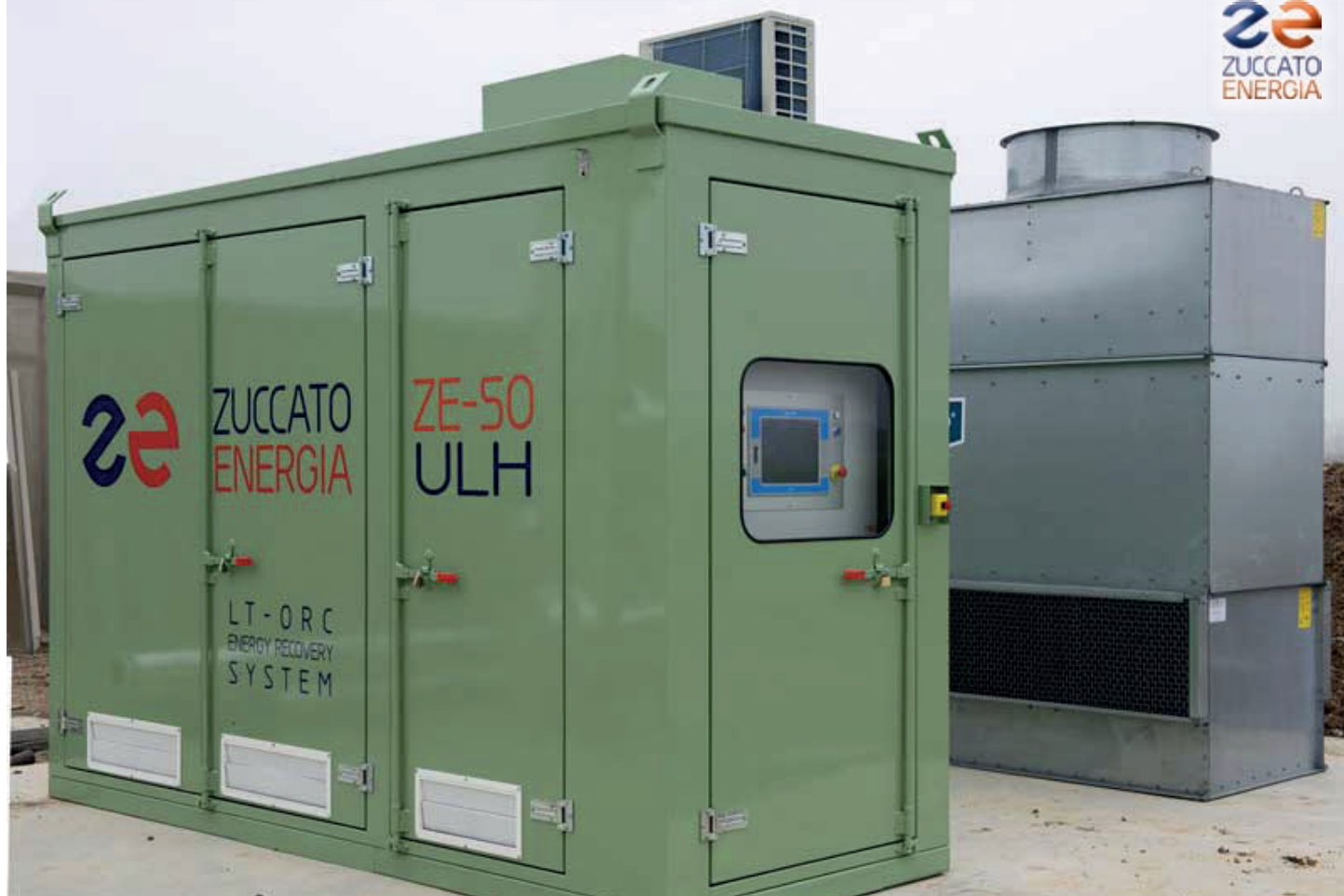
Lombardy 01 / Mantua: The weatherproof containerized ORC module and, behind it, the cooling tower.
