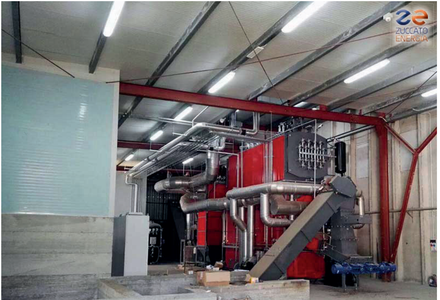
Calabria 01 / Cosenza : The boiler seen from the biomass loading side
