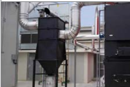
The dust trap. Wood burns cleanly, requiring only minimal ue g as treatment
