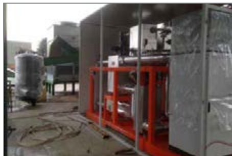
The skid during installation in the soundproof enclosure.
