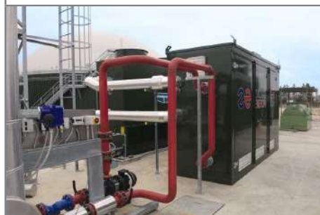
The ORC module (connectors side).
