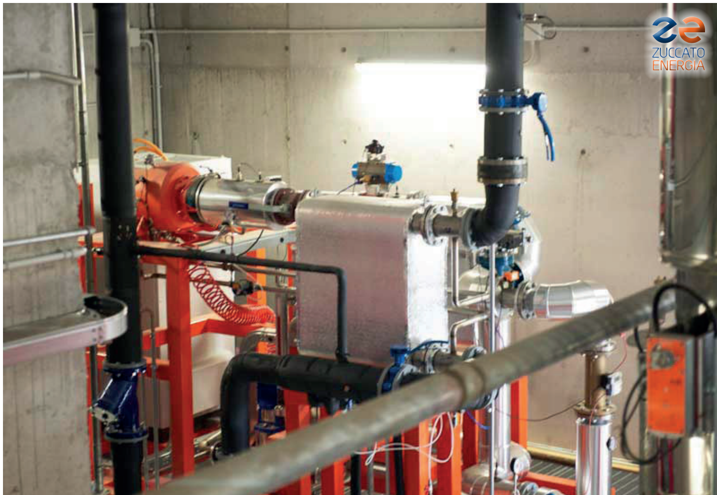
Veneto 03: The ZE-50-ULH low-temperature ORC module seen from above
