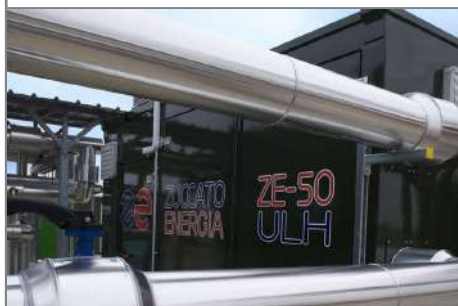
The ORC module (back side).
