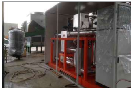
The ZE-100-LT ORC module being installed in its noise-absorbing enclosure.
