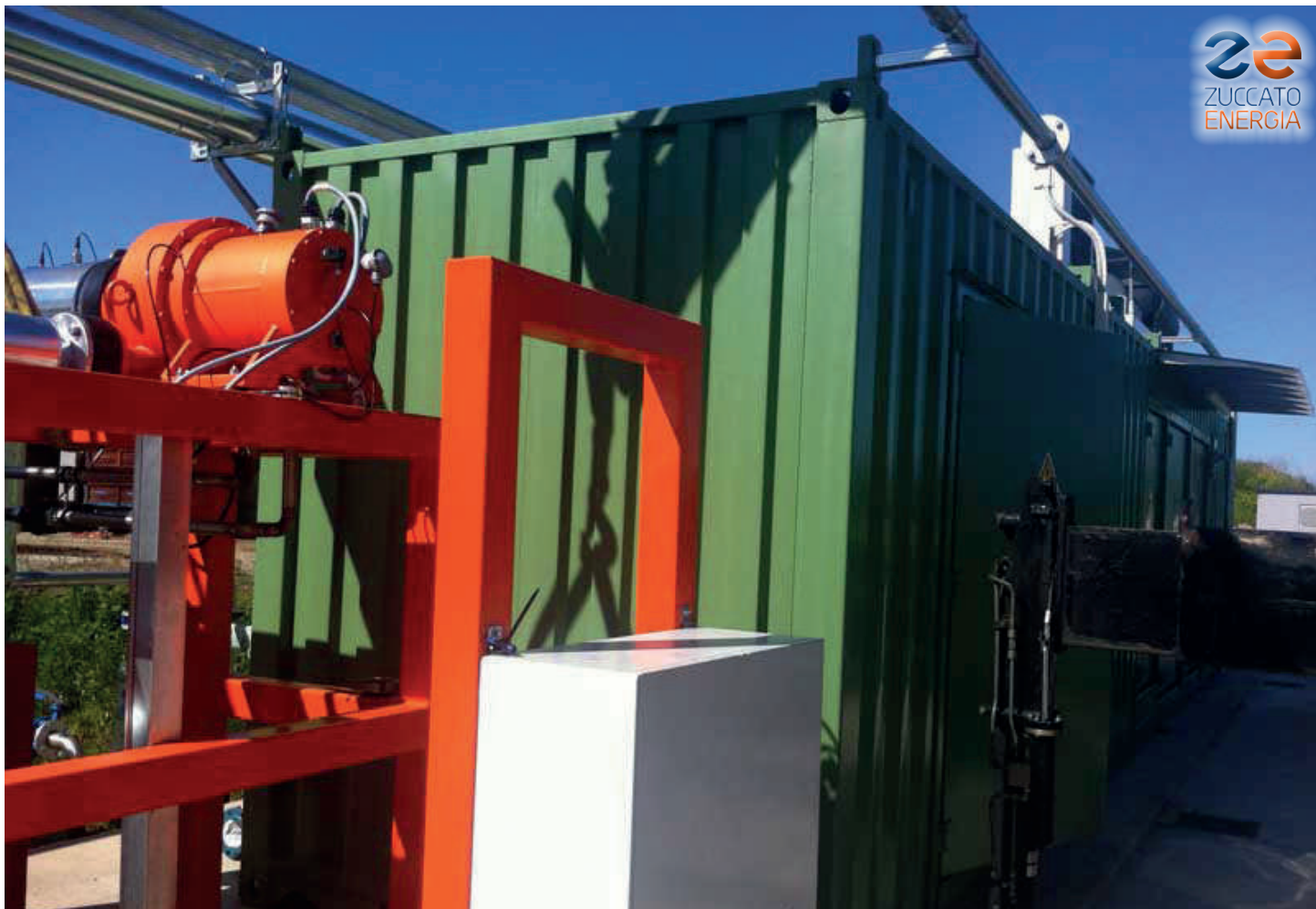
Veneto 02: The ORC module (orange) with its contact box (white) and the containerized control room (green)
