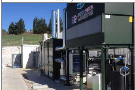
Behind the cooling tower, the ORC module, in its weatherproof containerized enclosure.
