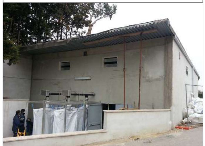
The gasifiers housing: in the foreground, its ash disposal system.
