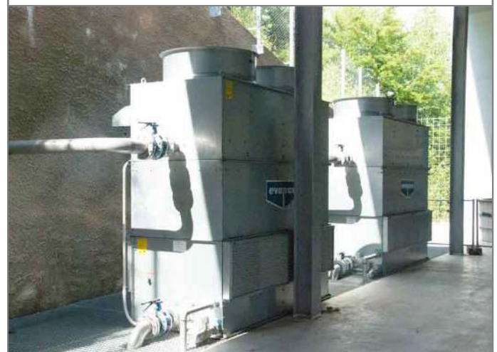
The cooling towers, installed behind the building.
