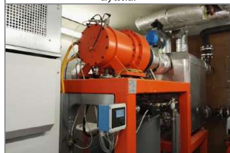
The ZE-50-ULH ORC skid in its place inside the prefabricated shed.
