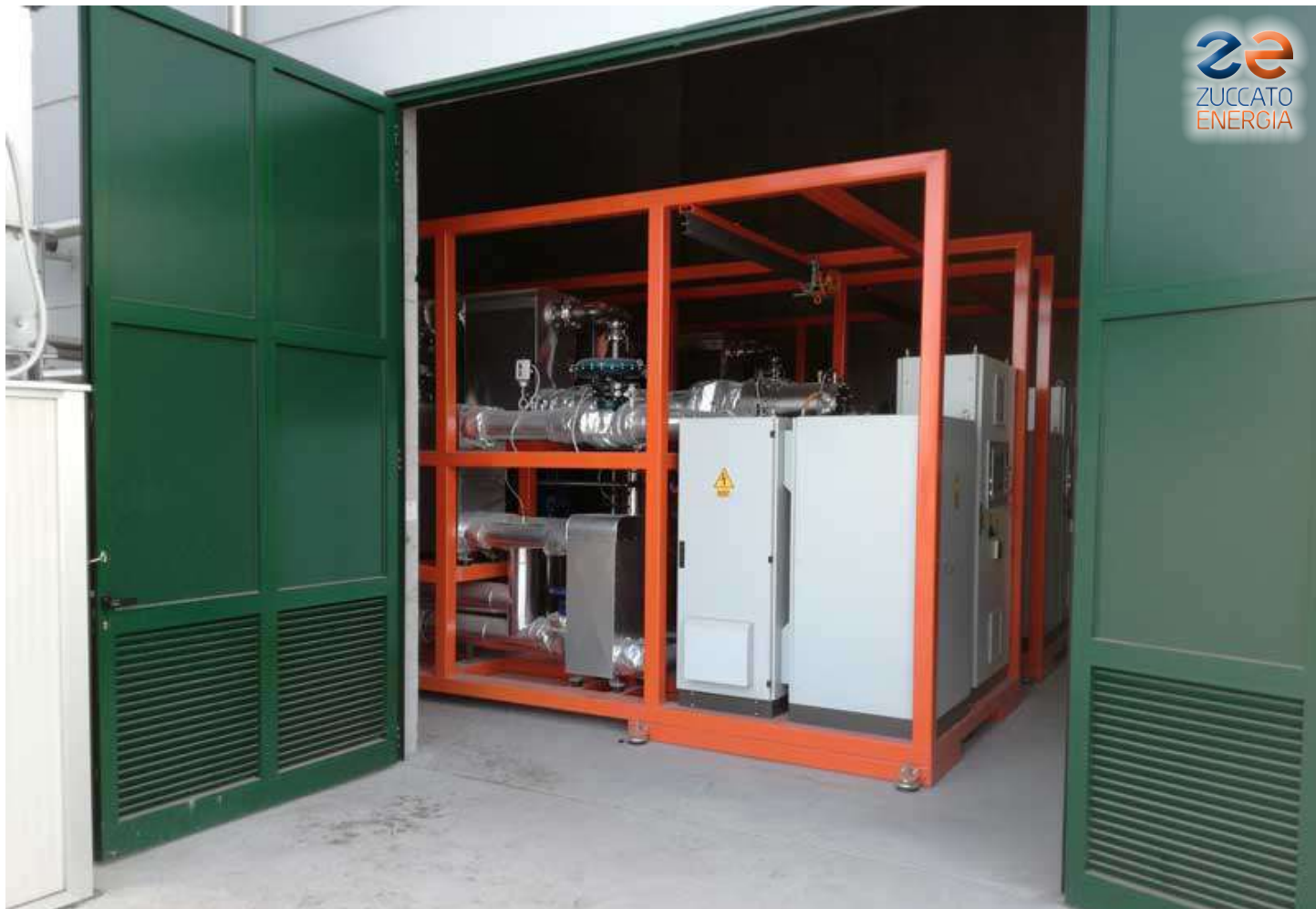
Veneto 04: The two skid-mounted ZE-100-LT Organic Rankine Cycle modules in their room
