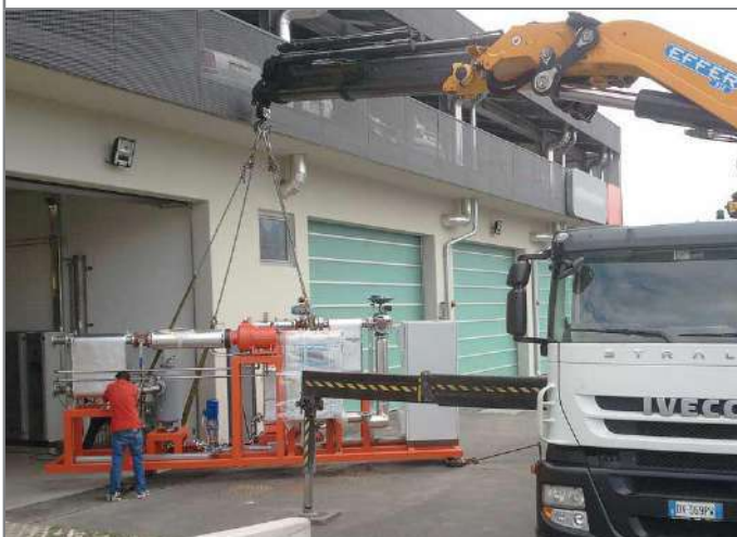
The ZE-50-ULH LT-ORC skid being unloaded.
