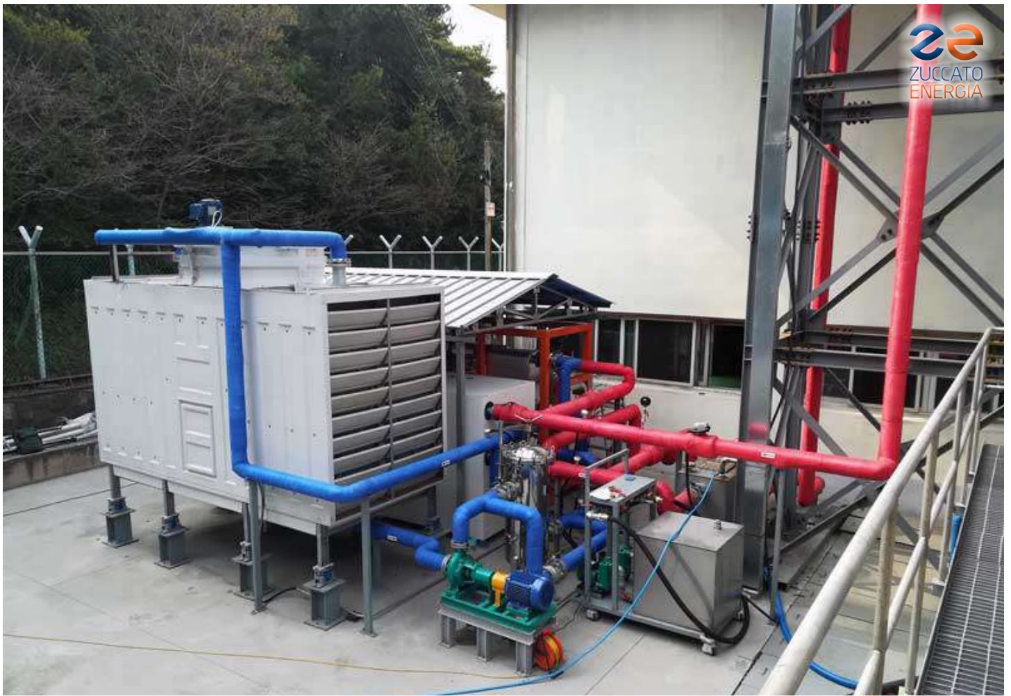
Korea 01 : The cooling tower and the awning hosting the ZE-40-ULH organic Rankine cycle power generation module.
