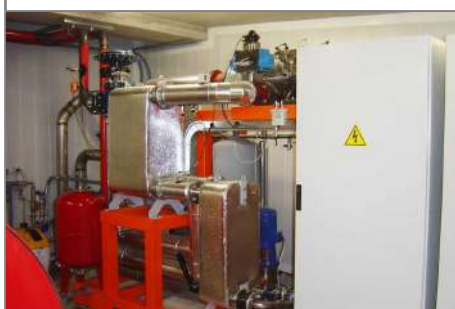
The ZE-40-ULH ORC module in detail.
