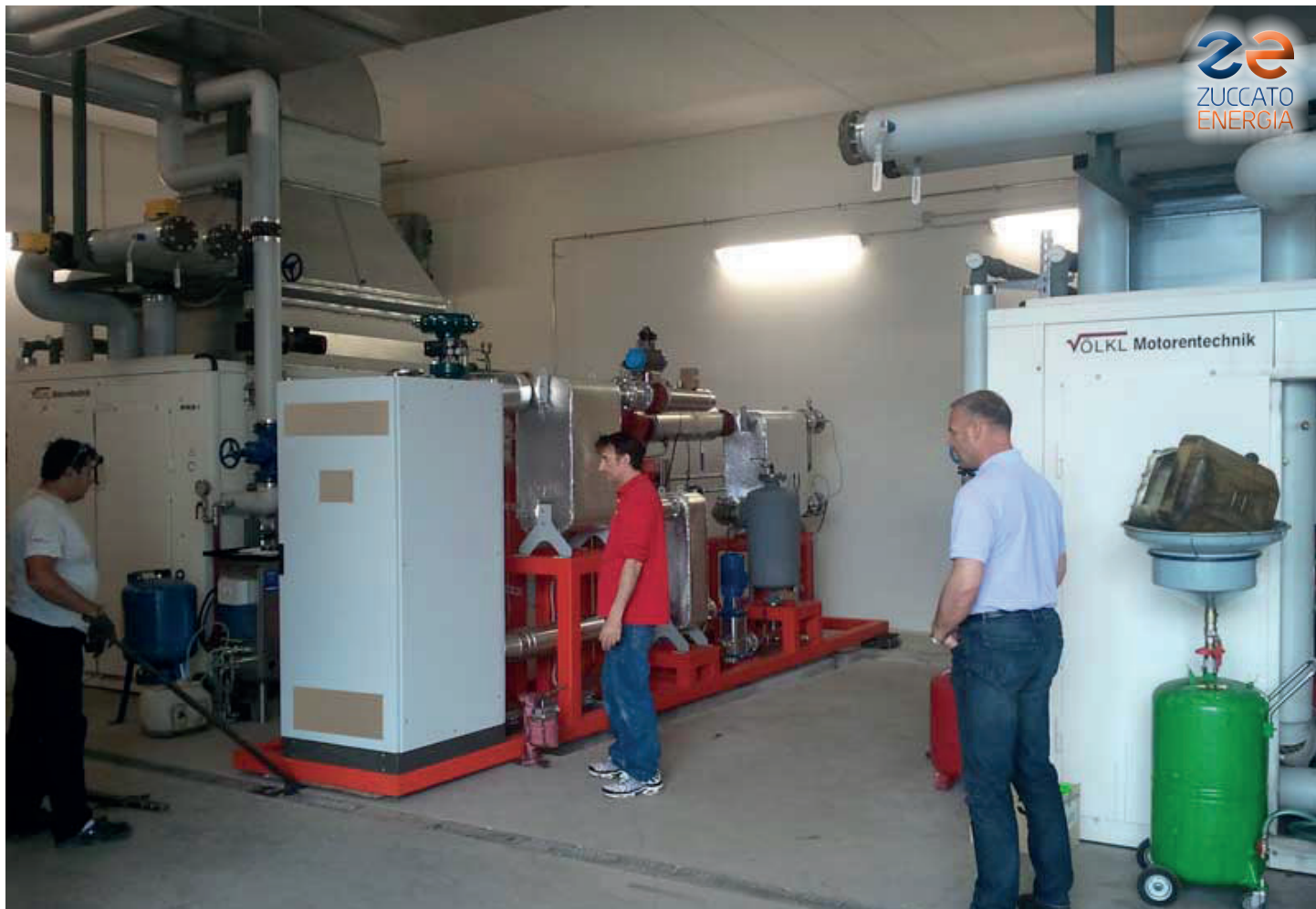
Alto Adige 04 : The first LT-ORC skid being installed
