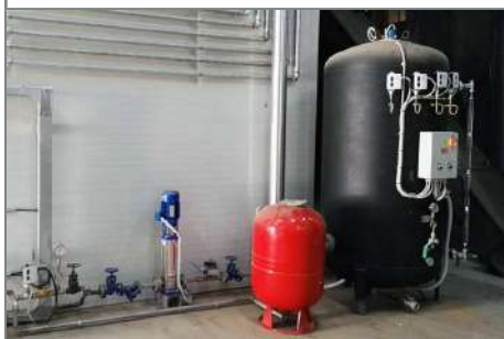
The vector fluid expansion vessel.
