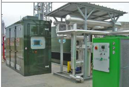
The ORC module (control panel side).
