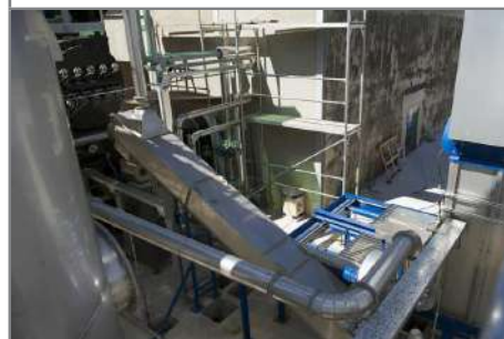
General view of the fuel loading screw.
