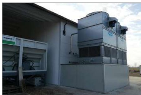
The evaporative cooling tower.
