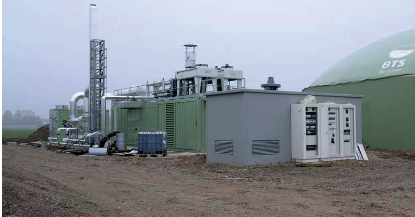
Lombardy 01: A general view of the fermenters, the engines and the containerized ZE-50-ULH ORC module
