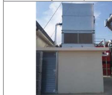
The cooling tower which dissipates the excess heat of the ORC condensation stage.
