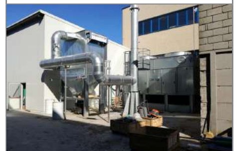
L to R: the bag filter for flue gases, the chimney and the cooling tower.
