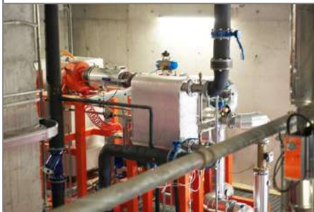
The ZE-50-ULH ORC system seen from above.
