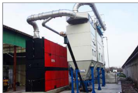
The boiler (L) and the exhaust treatment system.
