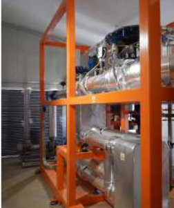
The ZE-175-LT ORC module in its skid, seen from the left side.
