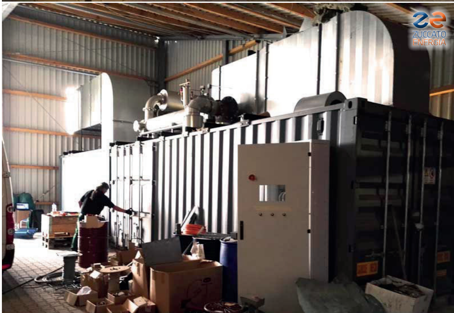
Germany 02: The container hosting the biogas-fueled MAN genset
