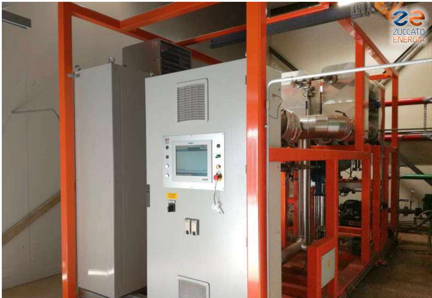
Lombardia 03: The ZE-150-LT organic Rankine cycle power generation module, seen from the control panel side
