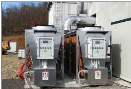
A detail of the dry cooler control panels.
