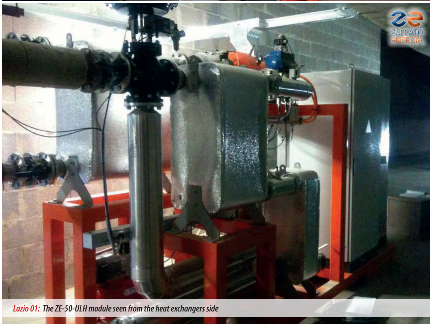
Lazio 01: The ZE-50-ULH ORC module in its underground space below one of the cinema theaters
