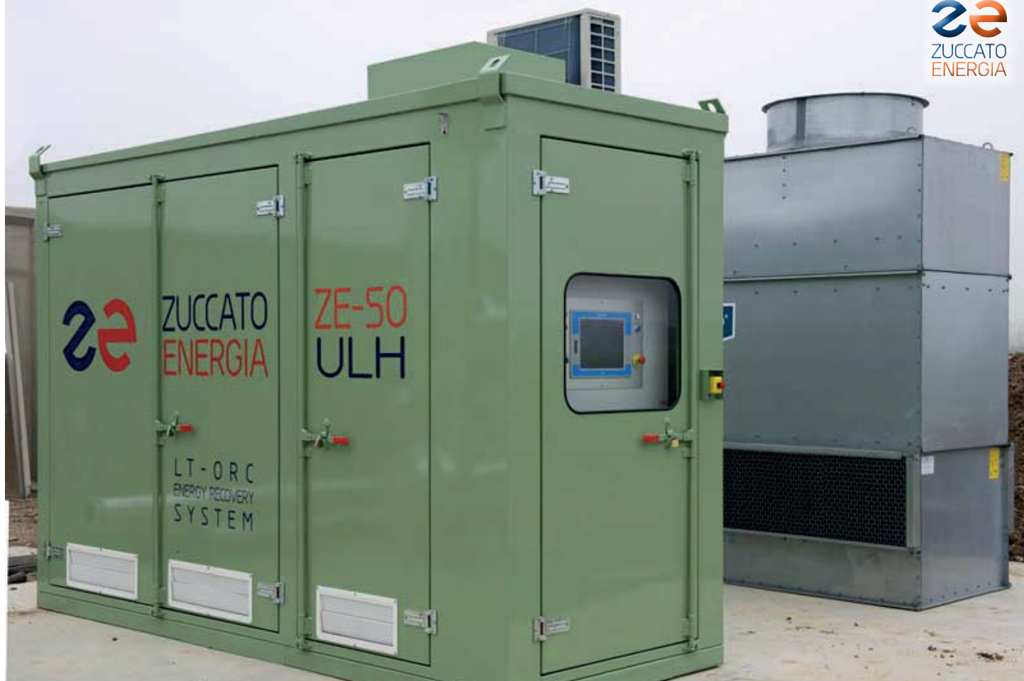
Lombardy 01: The containerized, weatherproof ZE-50-ULH ORC module; in the background, the cooling tower
