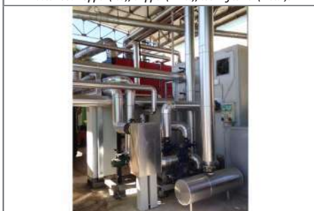
A detail of the fully insulated thermal connections to the boiler.
