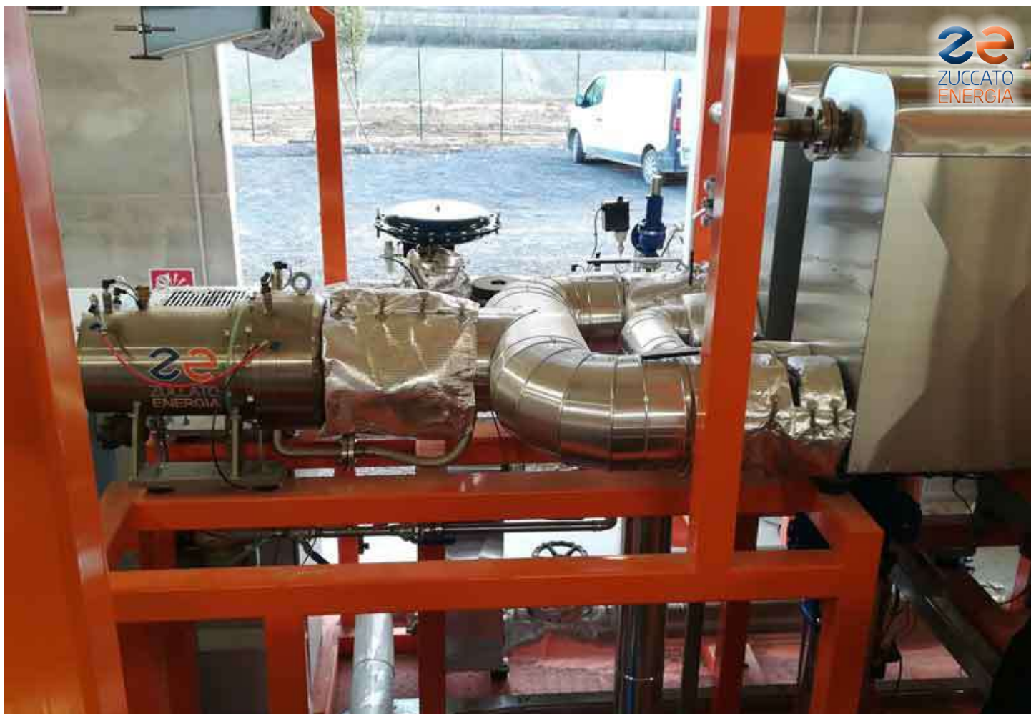
Umbria 01: A detail of one of the two ZE-100-LT ORC modules in their own room
