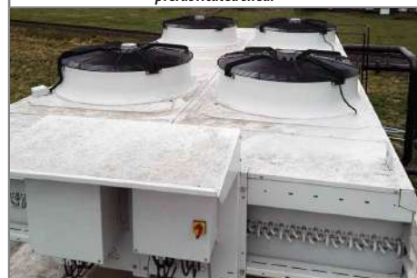
A close-up of the dry coolers on the roof.
