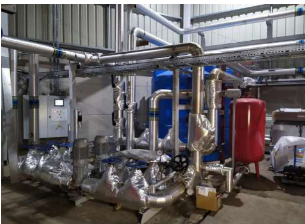
Boiler preheating system and superheated water at the ORC.
