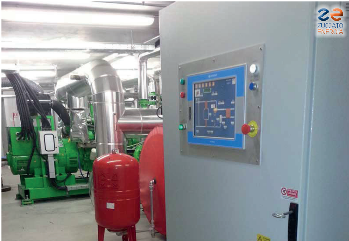
Aosta Valley 01: A general view of the underground boiler room with engines (green), heat buffer (red) and ORC module
