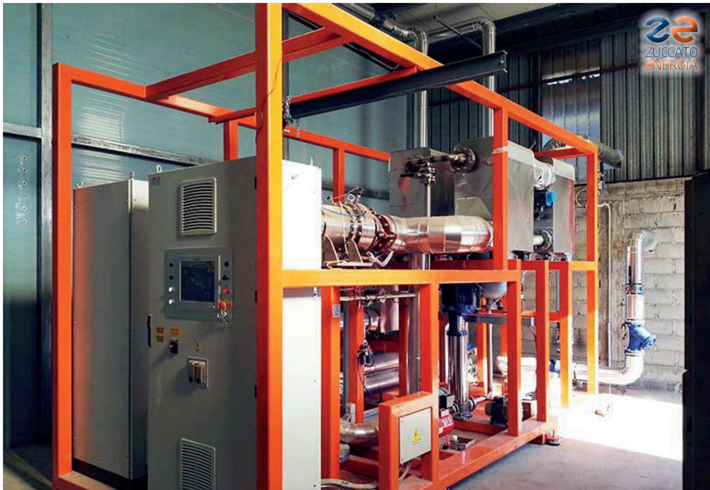
Calabria 01 : The ZE-175-LT ORC module in its place, seen from the control panel side
