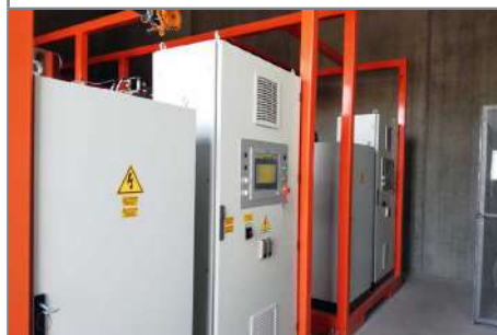
The control panels for the ORCs.
