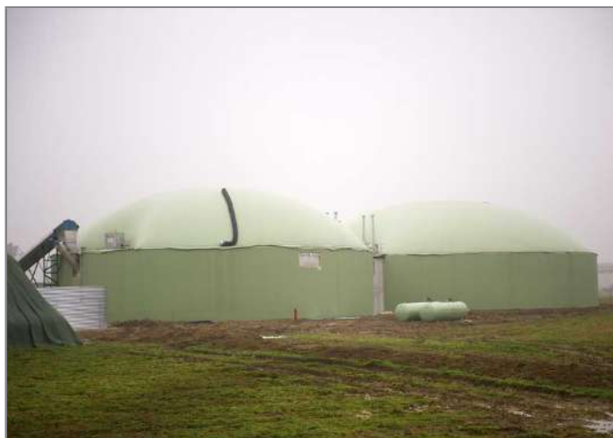
The main fermenter tanks.
