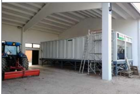
The biomass loading hopper.
