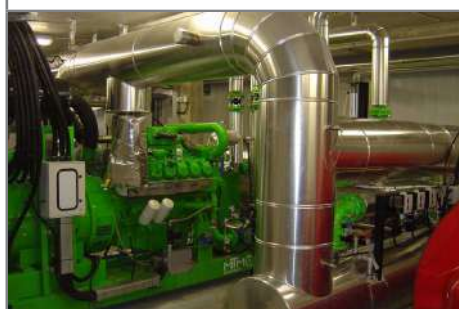
The vegetable-oil-fueled MAN 420 engine.
