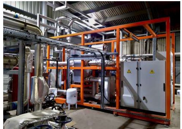
The ZE-105-CHP ORC module in place.
