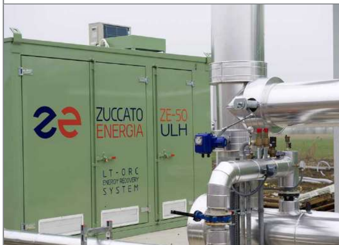
A side view of the ORC module container.
