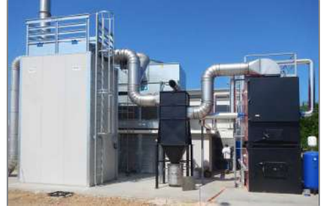
R to L: boiler, dust trap and flue gas treatment system.
