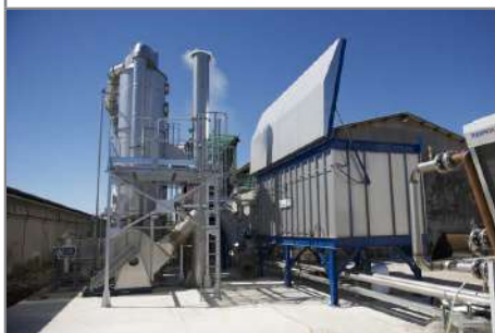
The fuel feeding hopper and the chimney.
