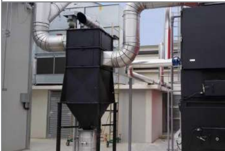
The dust trap. Wood burns cleanly, requiring only minimal flue gas treatment.
