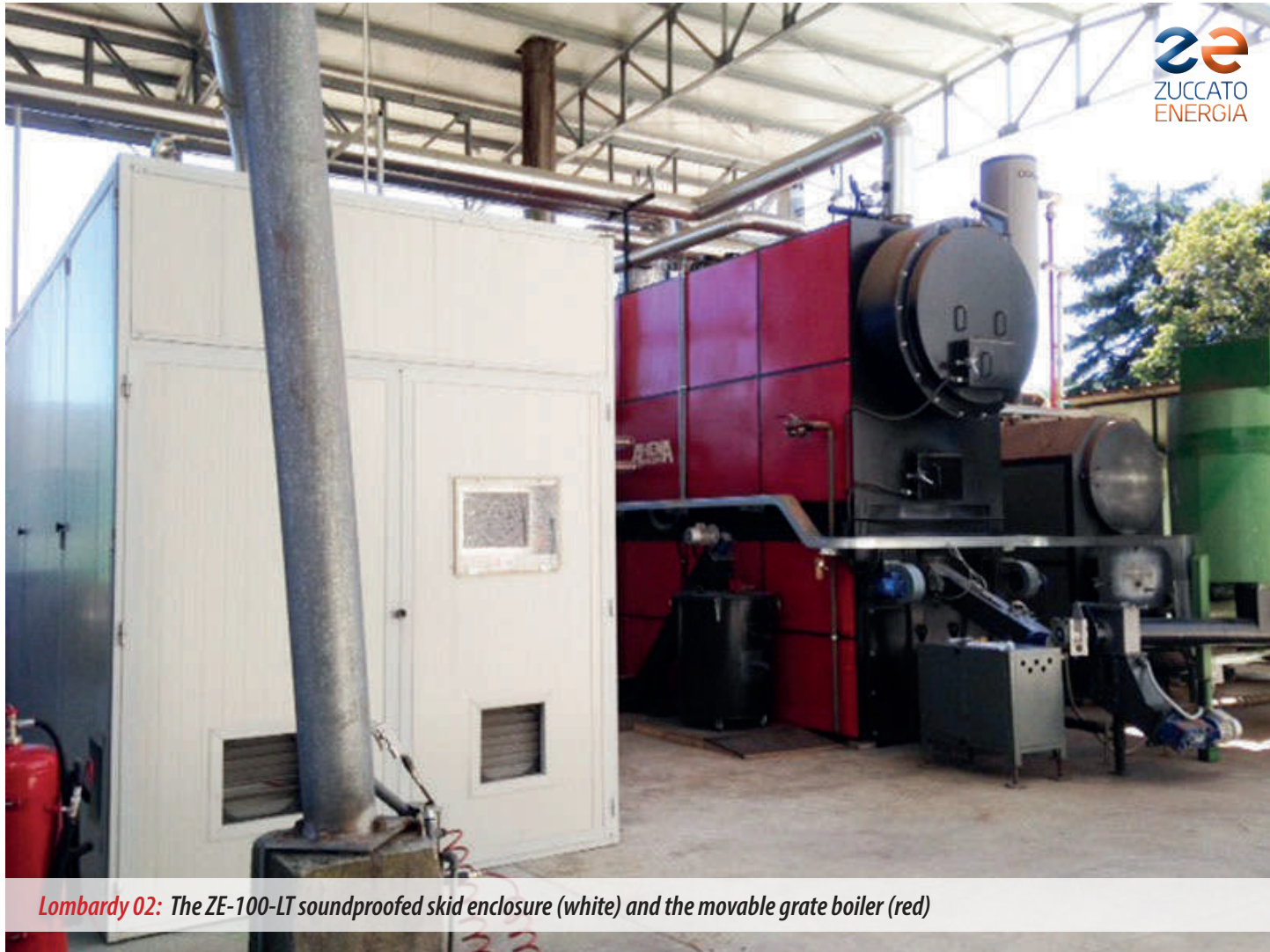
Lombardy 02: General view - L to R: ORC module enclosure (white), boiler (red), chip storage and conveyor (green)
