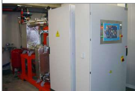
Overall view of the ZE-40-ULH ORC module.
