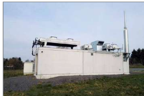
The east side of the plant. Note the roof-installed dry cooler.
