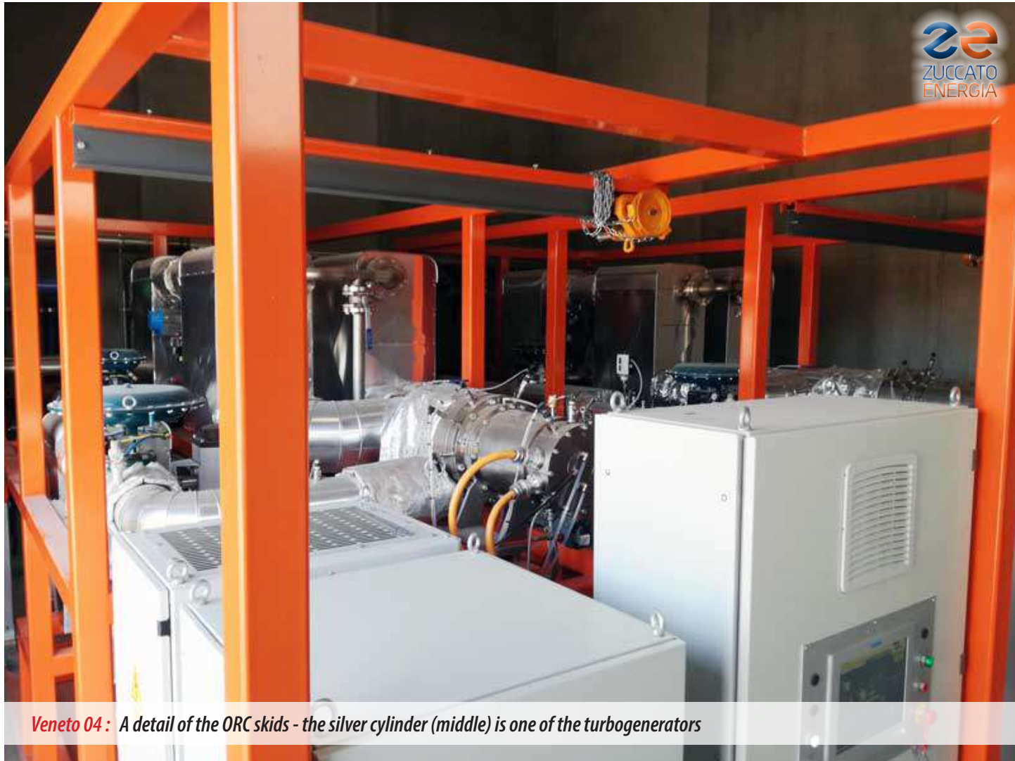
Veneto 04: The two skid-mounted ZE-100-LT Organic Rankine Cycle modules in their room
