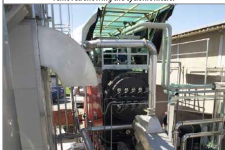
Detail of the loading screw and the burner.
