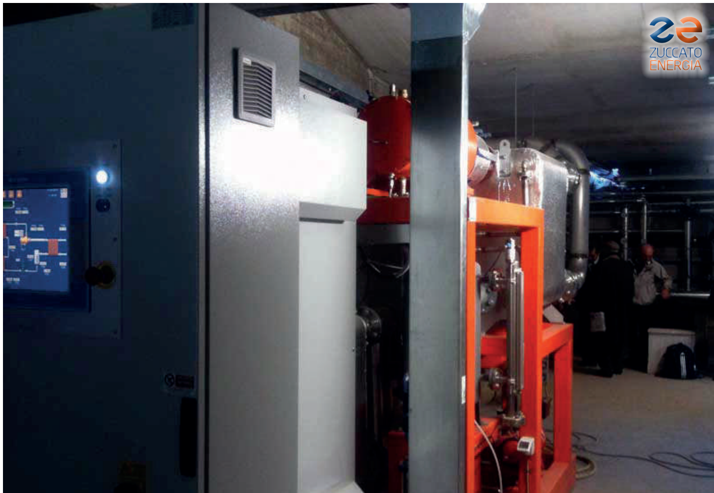
Lazio 01: The ZE-50-ULH ORC module in its underground space below one of the cinema theaters
