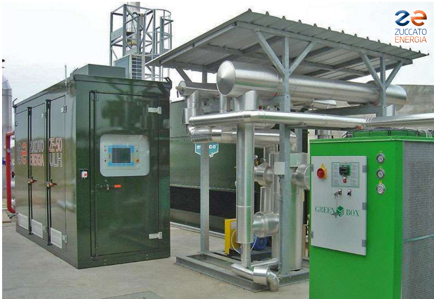
Veneto 01: The ORC module (control panel side)
