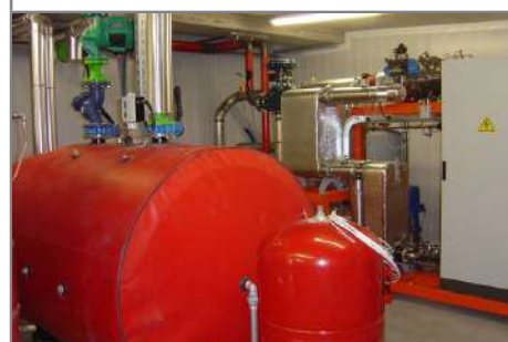
The "puffer" (thermal flywheel) and the ORC module.
