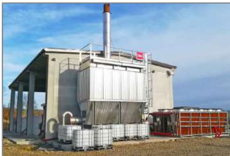
Flue gas treatment system and chimney. On the right, the dry cooler.
