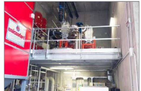
Overall view. Boilers are below, ORC plant in on mezzanine.
