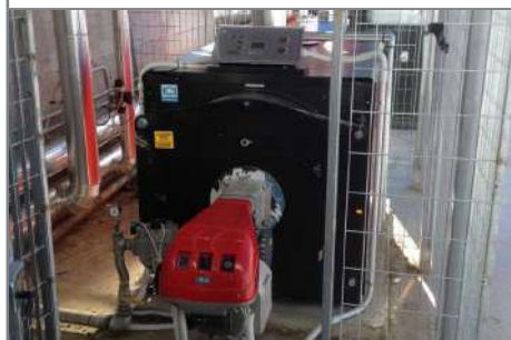
The ICI boiler which supplies most of the thermal energy for the plant.
