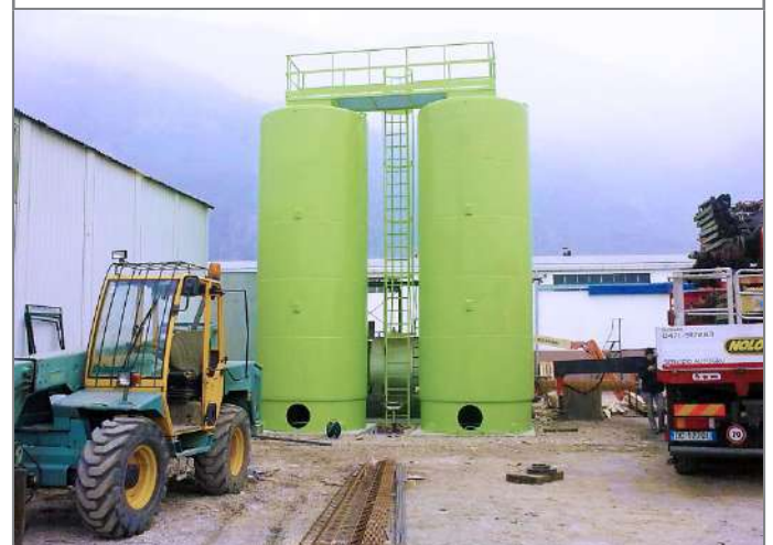
The vegetable oil reservoirs being installed.
