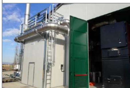
The flue gas treatment system and the boiler room.
