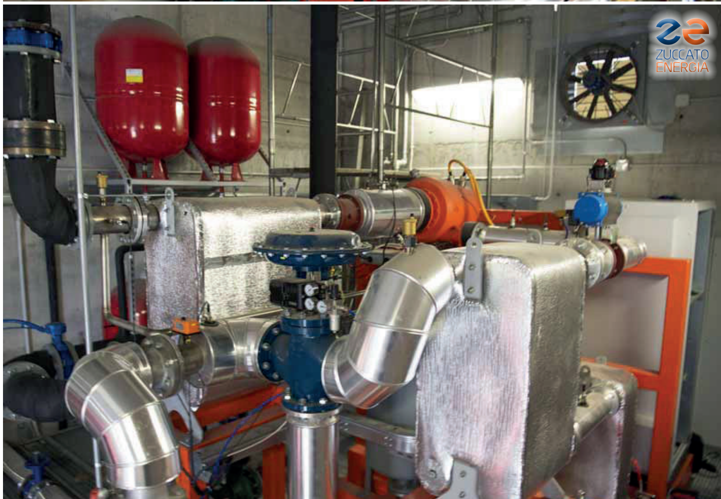
Veneto 03: A detail of the heat exchangers of the ZE-50-ULH low-temperature organic Rankine cycle module
