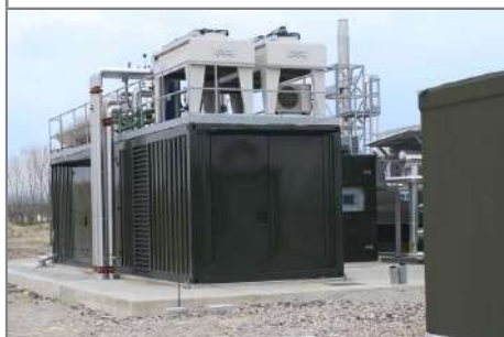
The container hosting the biogas-fueled engine.
