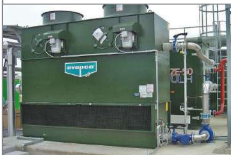
The cooling tower supplying the condenser.
