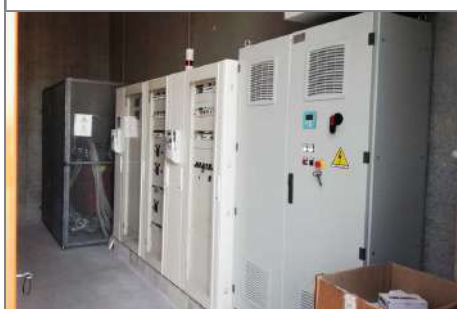
The mains grid interface panels.
