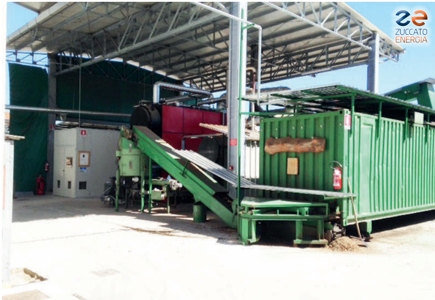
Lombardy 02: General view - L to R: ORC module enclosure (white), boiler (red), chip storage and conveyor (green)
