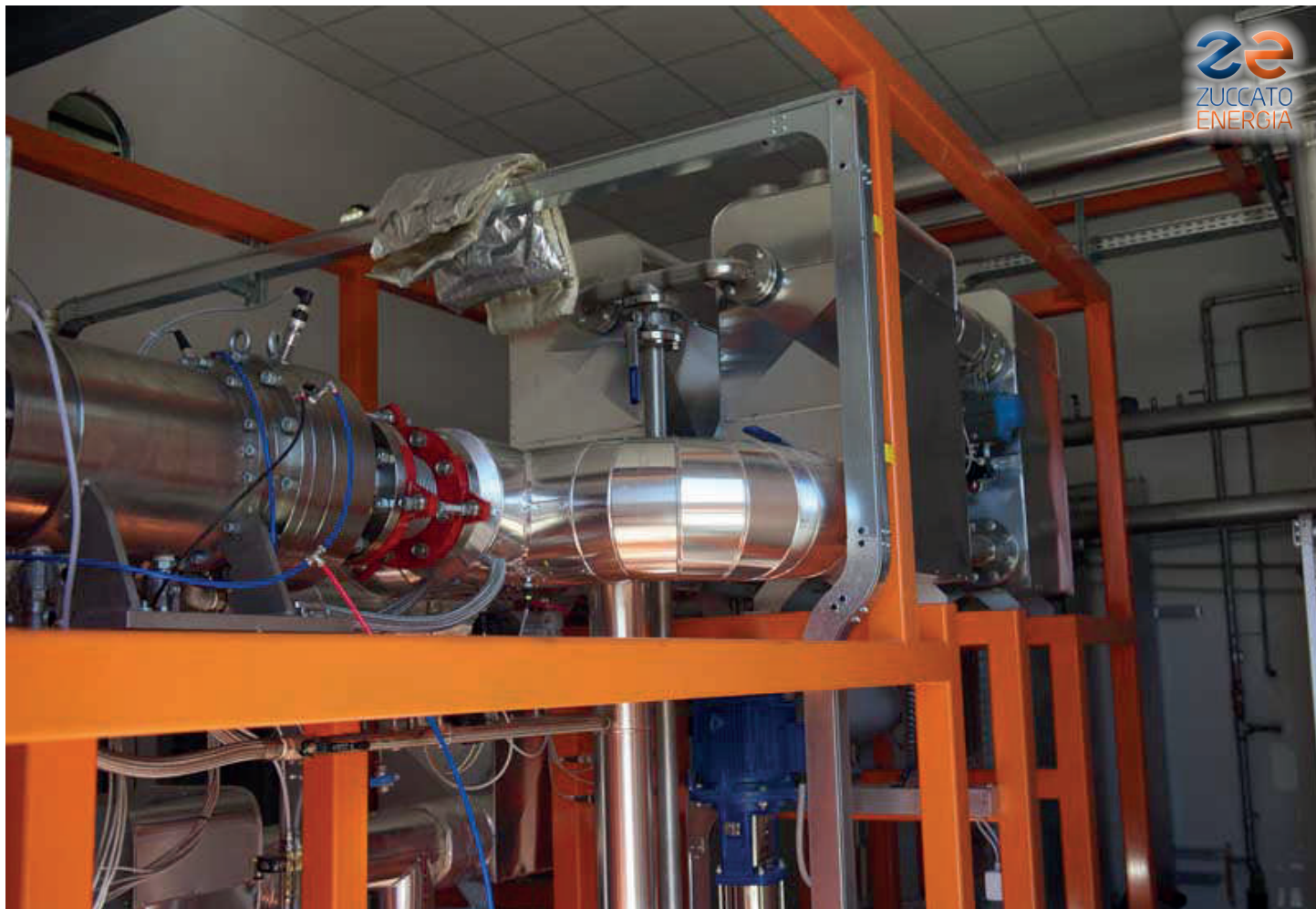
Friuli 01: A general view of the 150-kWe ORC module in its room
