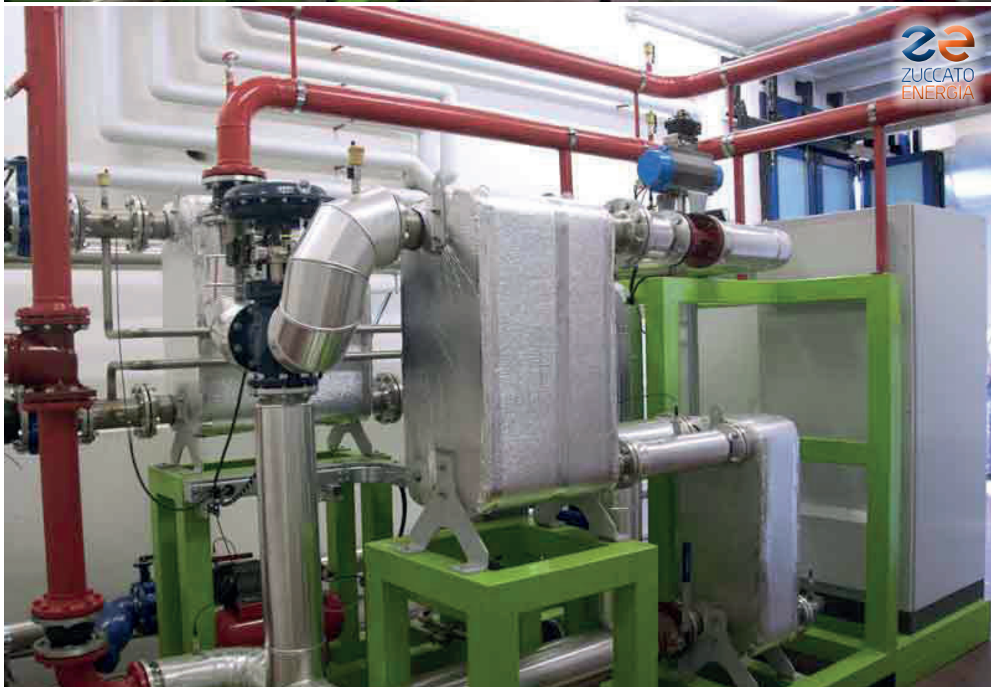
Alto Adige 02 : The ZE-50-ULH low-temperature ORC module in its place
