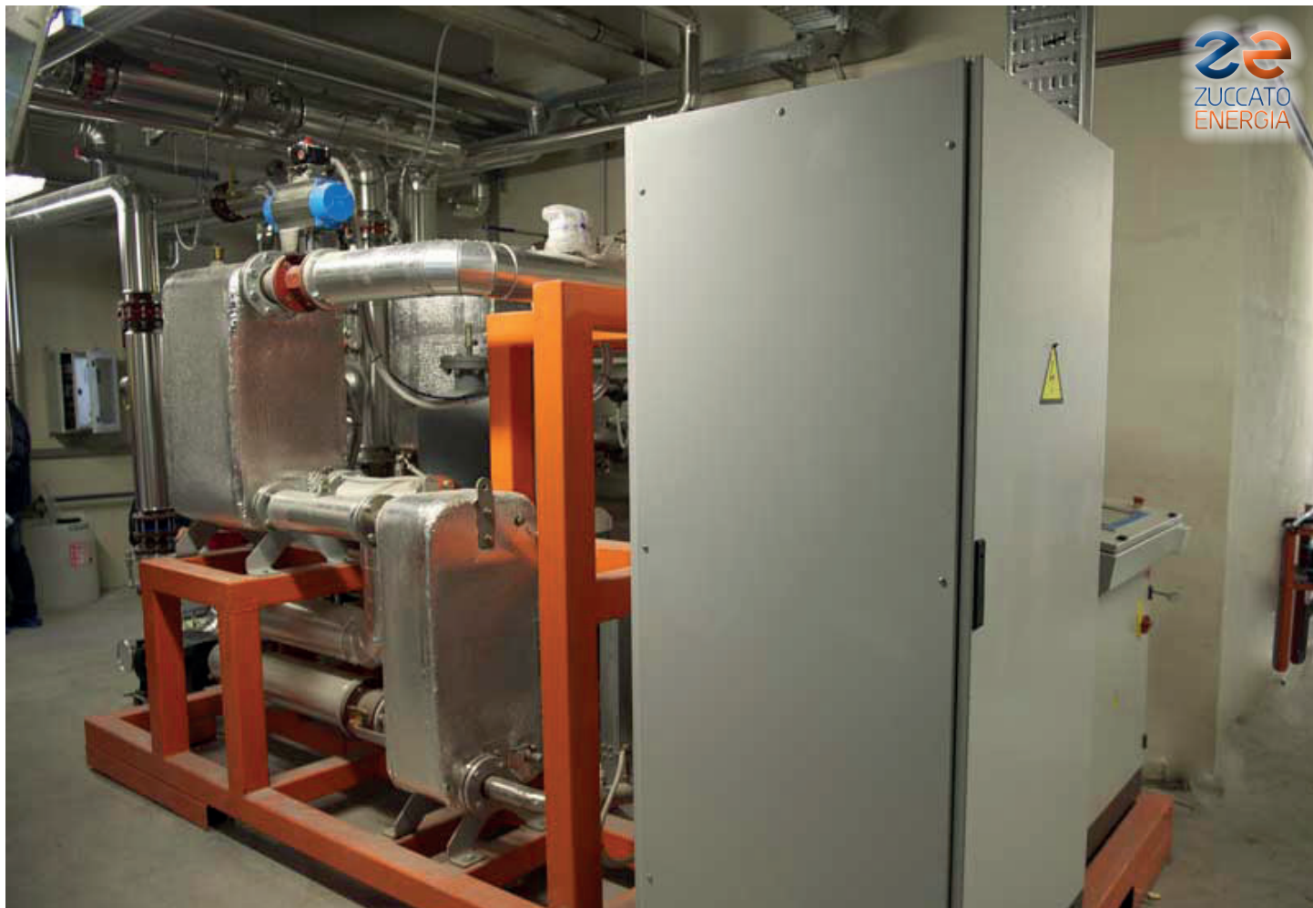
Alto Adige 03 : The ZE-50-ULH skid in place - seen from the side
