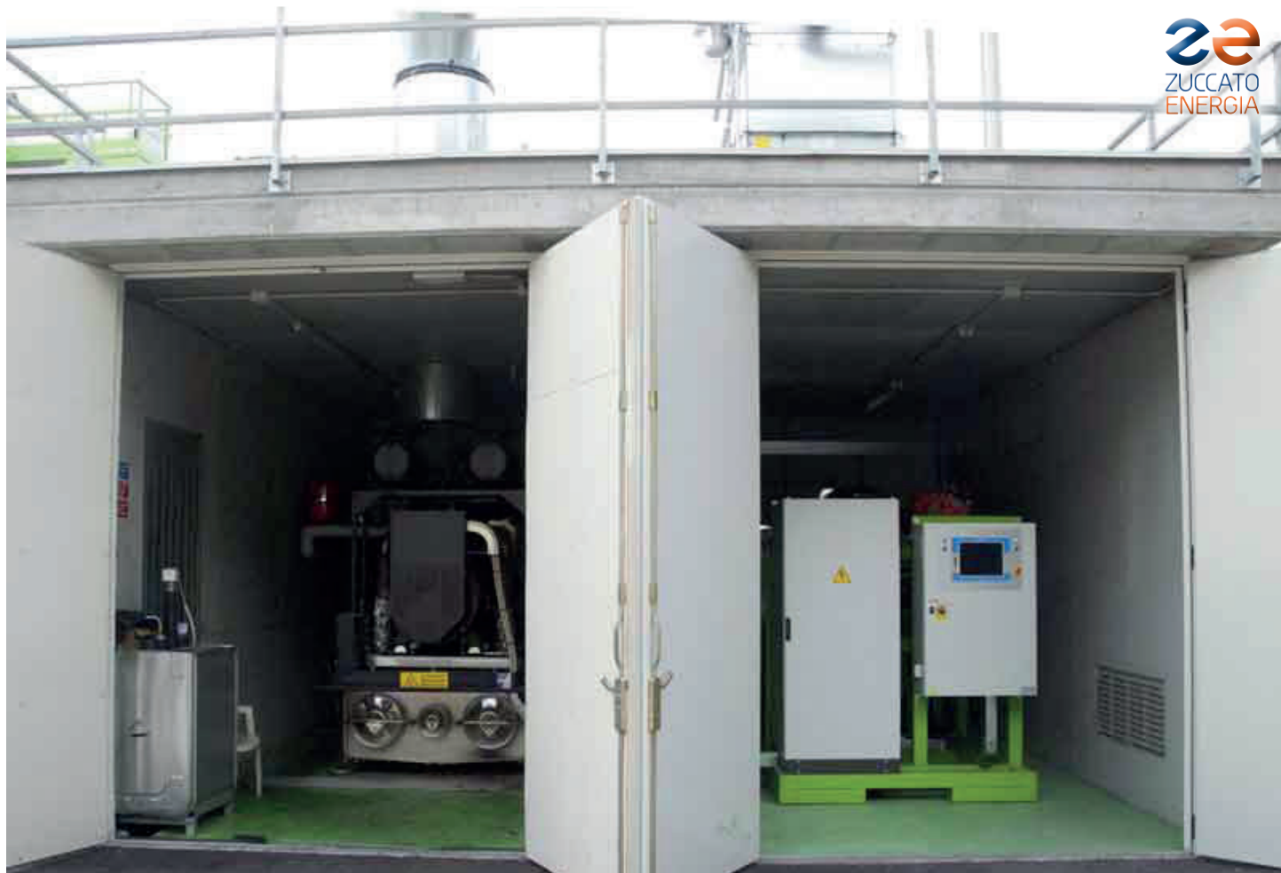
Alto Adige 01: The vegetable-oil-fueled engine (left) and the ZE-50-ULH low-temperature ORC module (right) in their shelter
