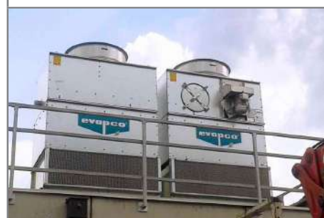
The cooling towers.
