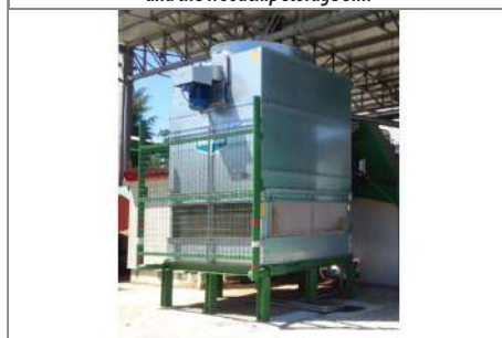
The cooling tower. A small one is sufficient, as residual heat is used to dry the wood chips.
