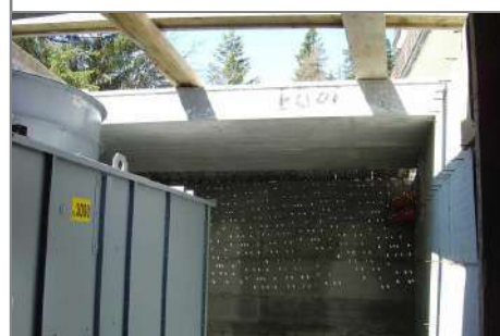
The cooling tower in its grid-ceiling room.
