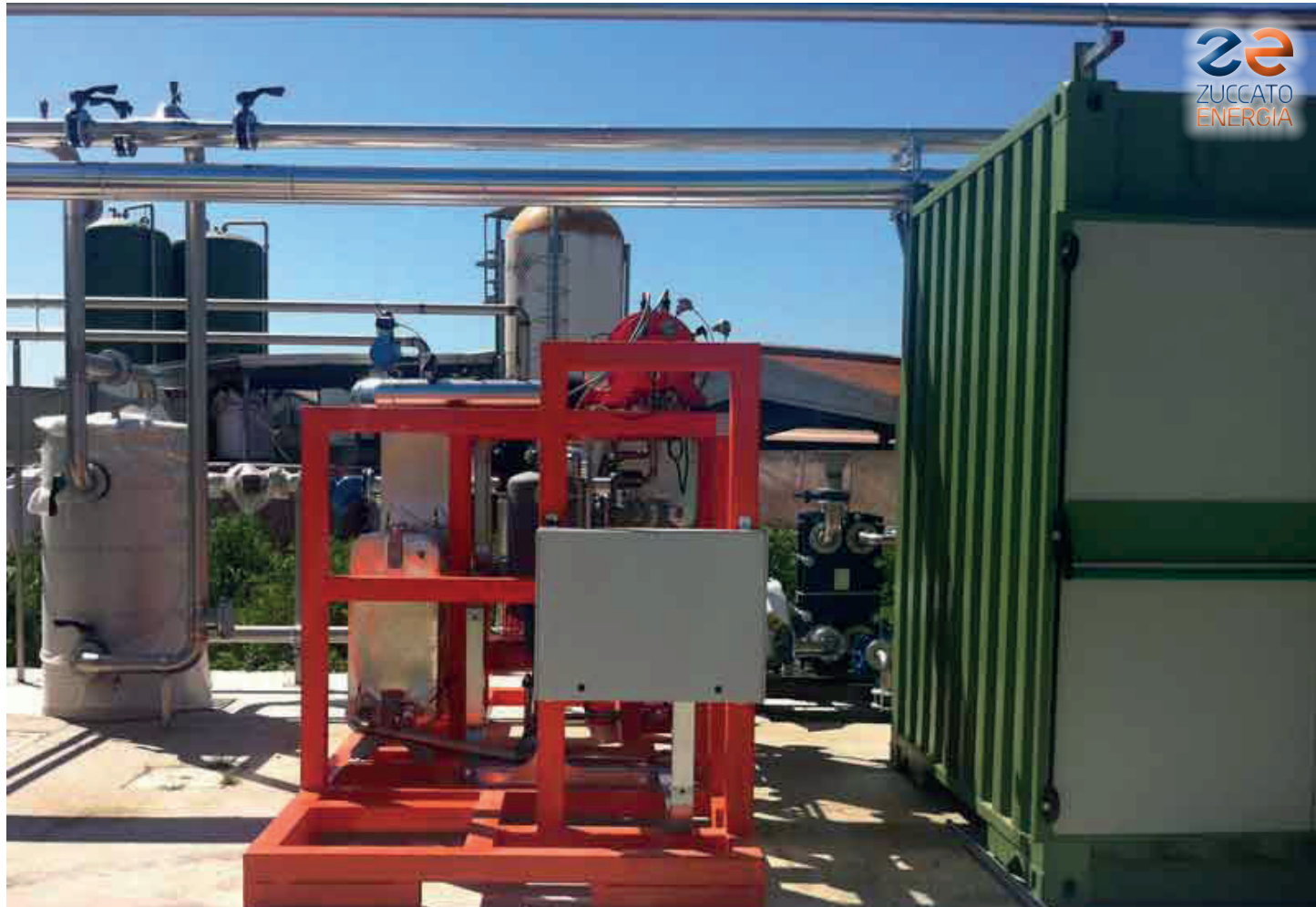
Veneto 02: The ZE-50-ULH low-temperature ORC installation seen from the front
