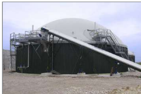
One of two fermenters with its load screw.
