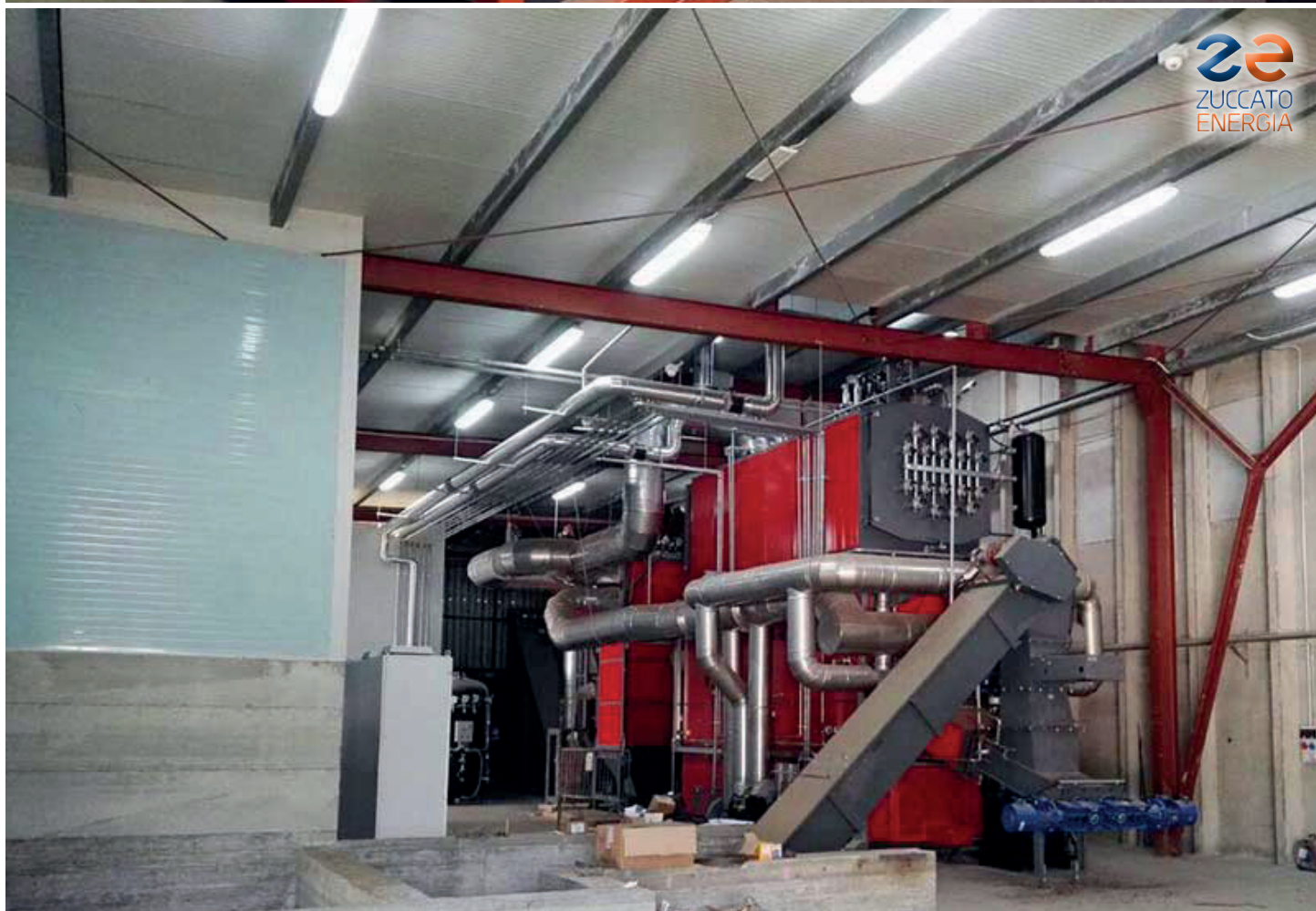
Calabria 01 : The boiler seen from the biomass loading side
