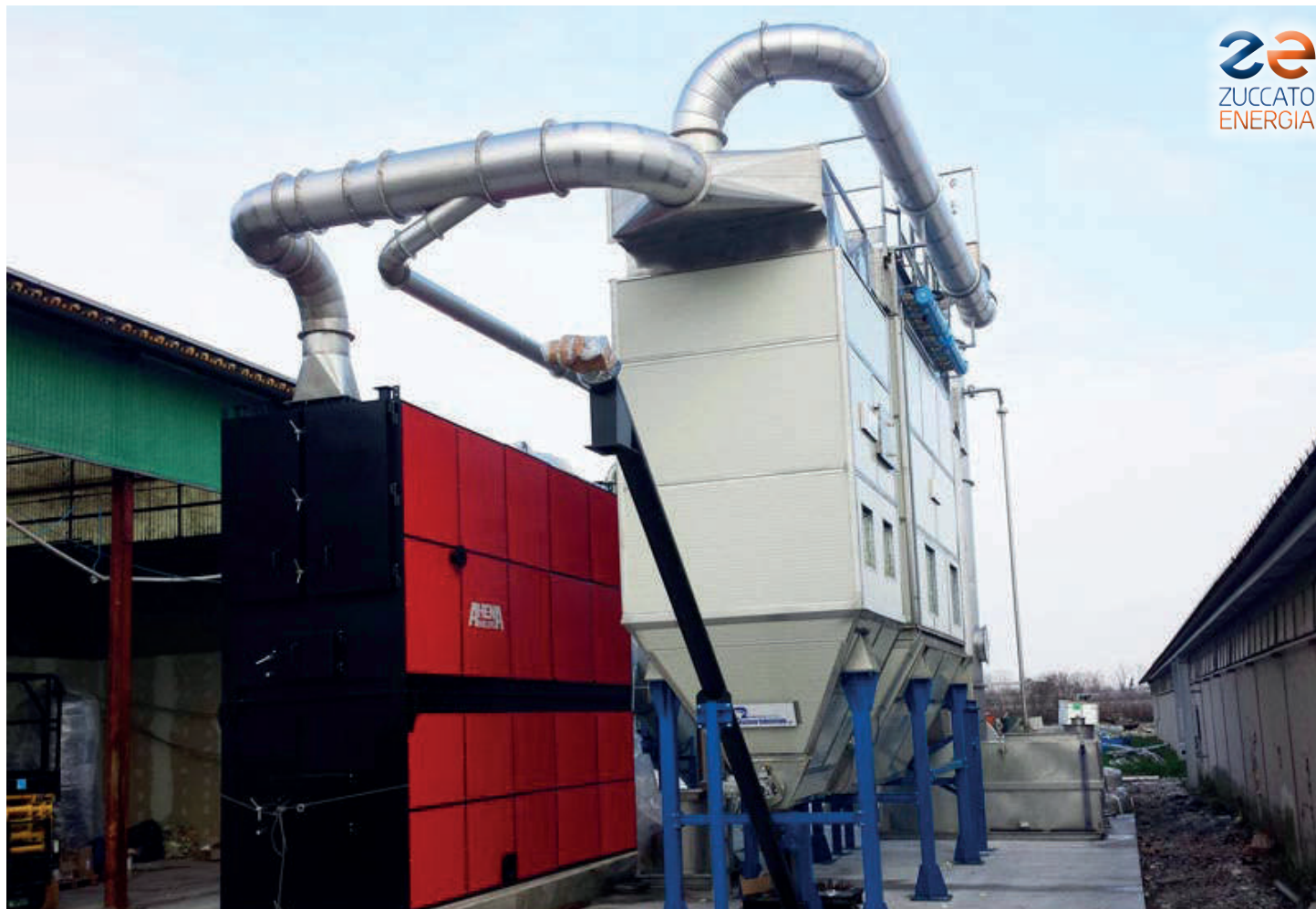
Friuli 01 : The boiler fueled by chicken dung (left) and the flue gas treatment system
