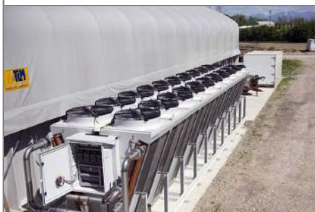
General view of the dry cooler.
