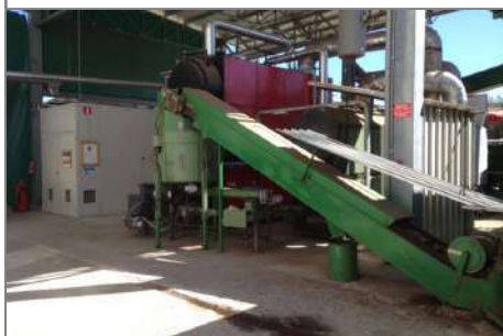
Detail of the storage-to-boiler fuel conveyor. Skid enclosure is in the background.
