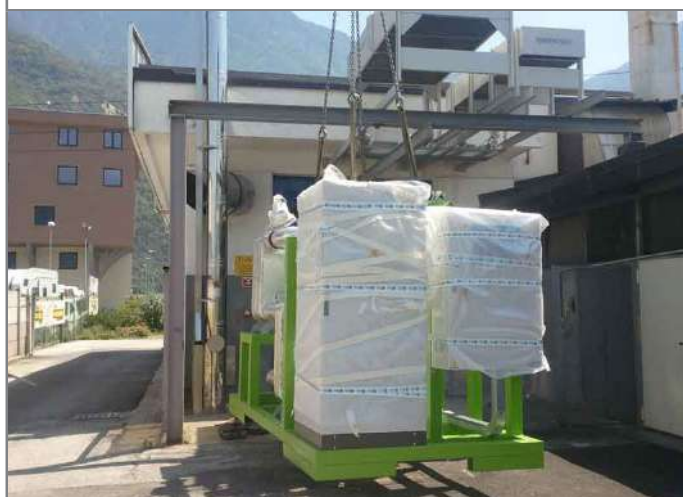
The LT - ORC skid being placed near its final location.
